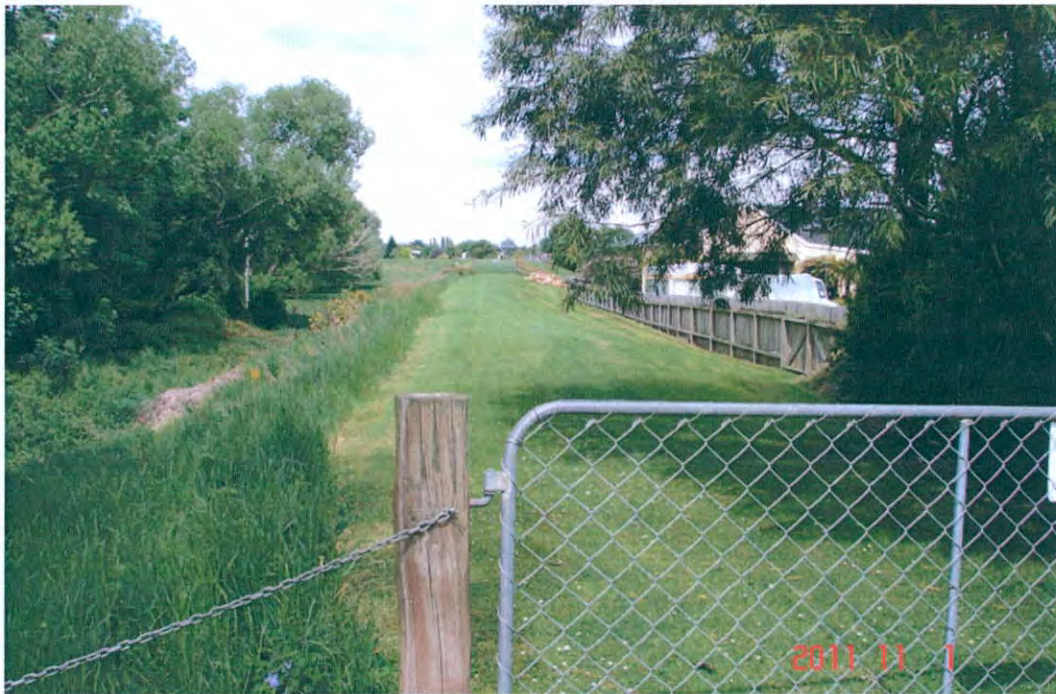
Figure 3.2: Photo of Taieri River right stopbank spillway section from upstream end on natural ground. 83m long extending to next gateway
