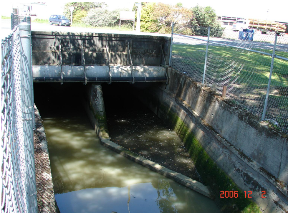
Photo 1: Photo of entrance to Opoho Creek culvert upstream of Ravensbourne Rd. Concrete wall level on right at ~RL102.6m
