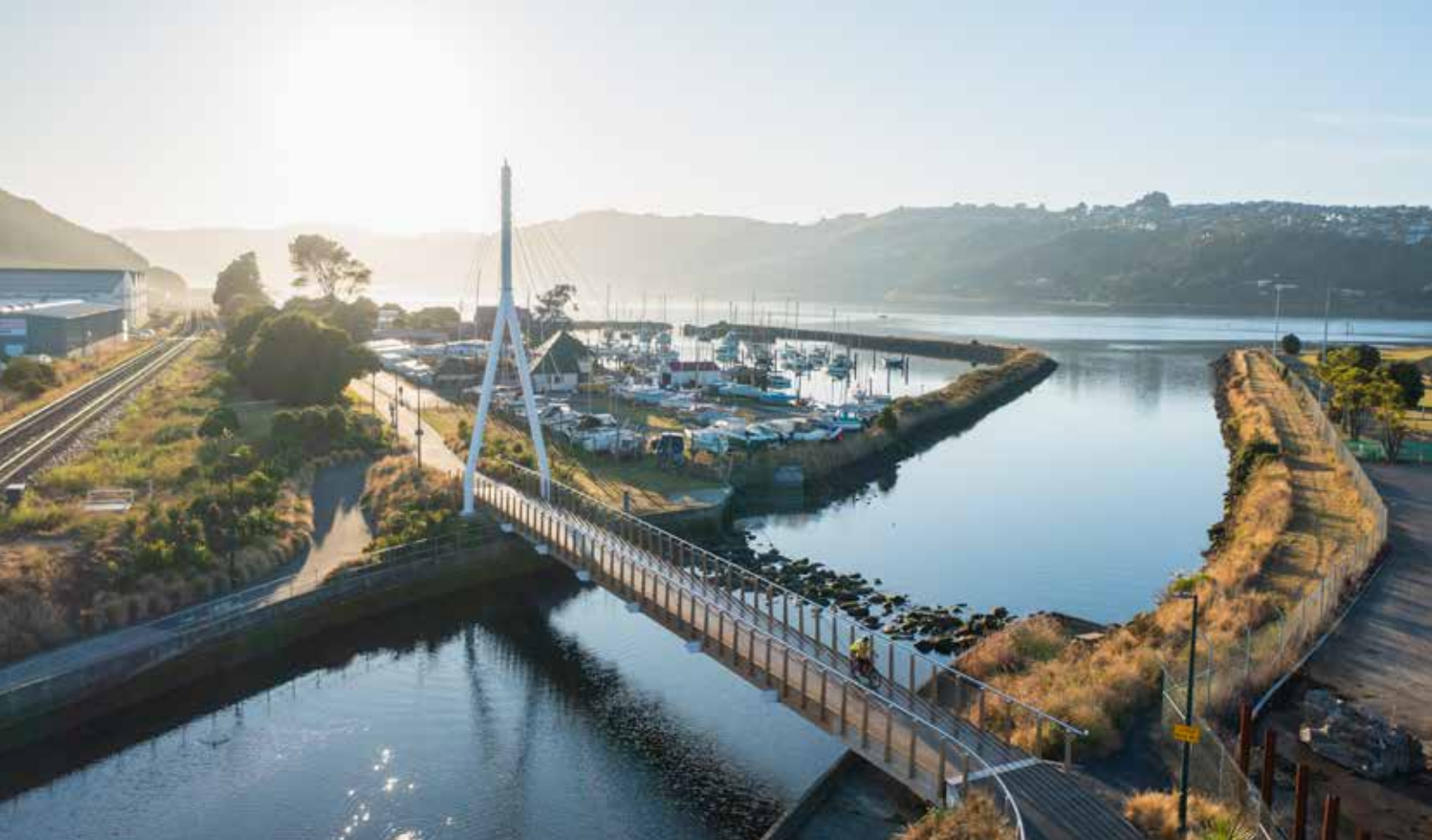
Figure 24: Te Aka Ōtākou – Bridge over Water of the Leith
