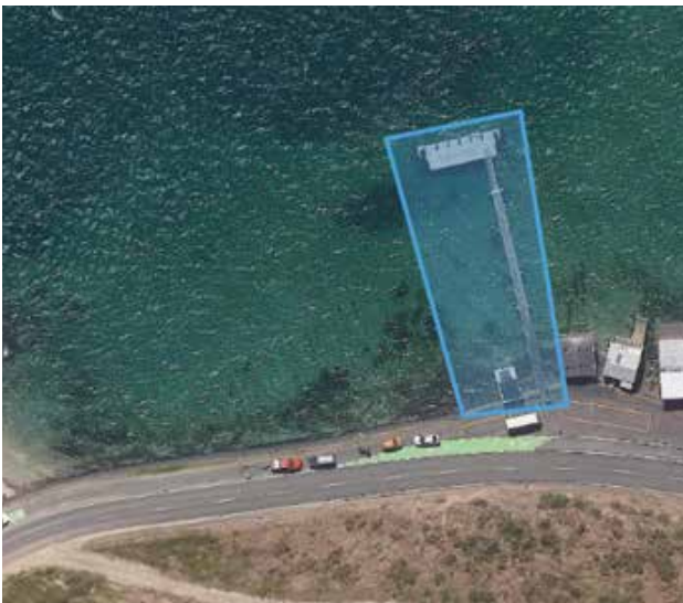
Figure 35: Wellers Rock Jetty location
