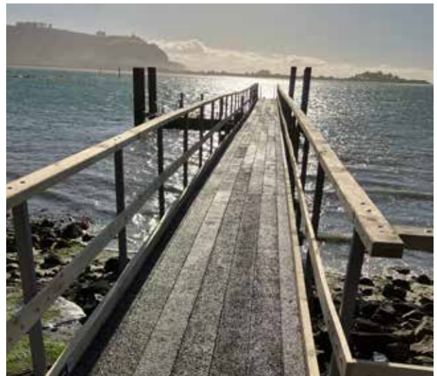
Figure 36: Wellers Rock (Te Umu Kuri) Jetty.
