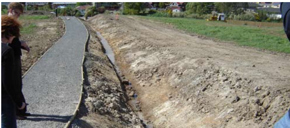
Work in progress - sustainable stormwater management initiative currently being constructed as part of a large residential development in Dunedin.
