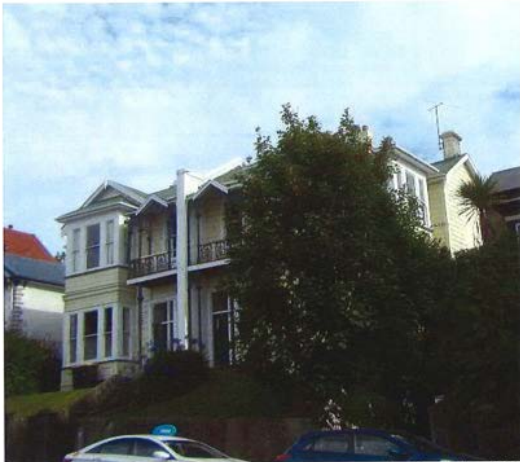
3. 332 & 330 High Street 21 February 2014. Photo by Peter Entwisle. The side bay of 330 is apparent at right. There is a matching one at 332.
