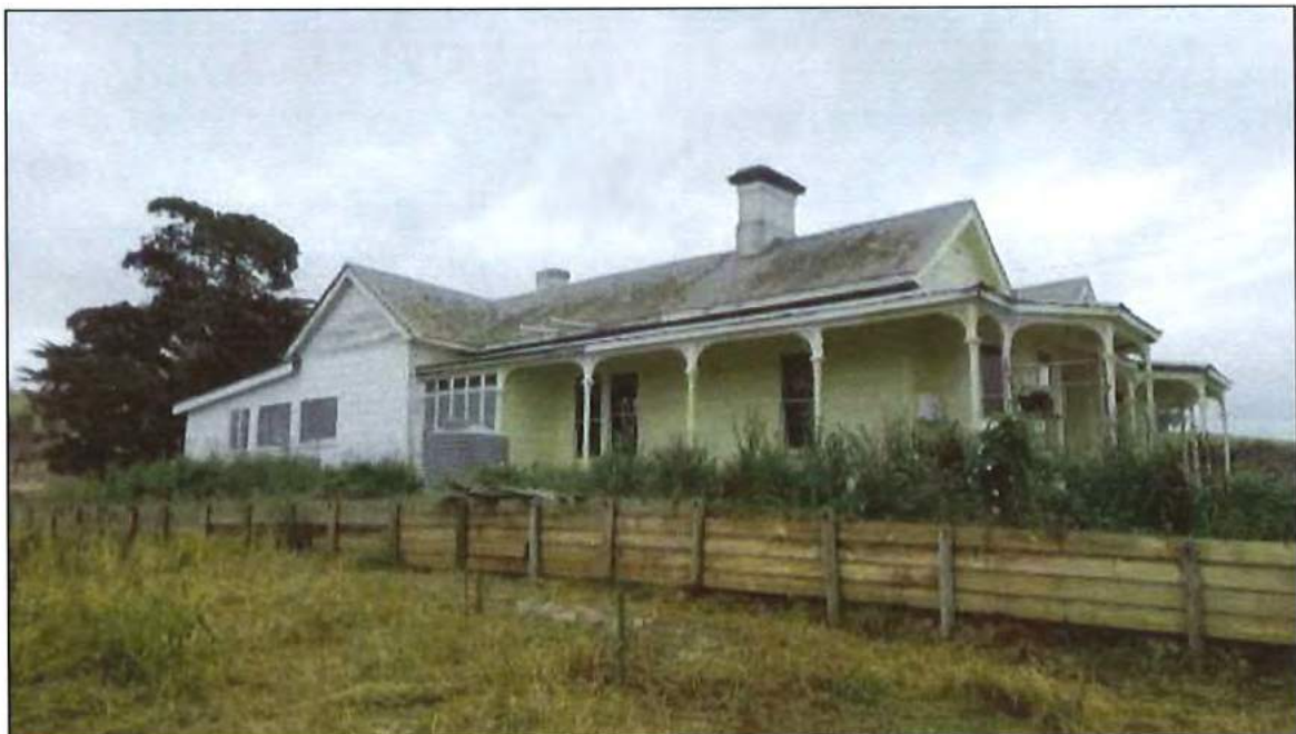
Figure 5. The house, looking north.
