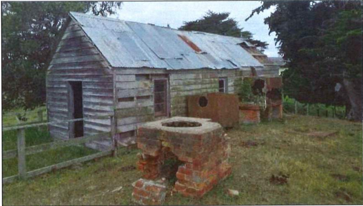
Figure 6. The store, looking east.
