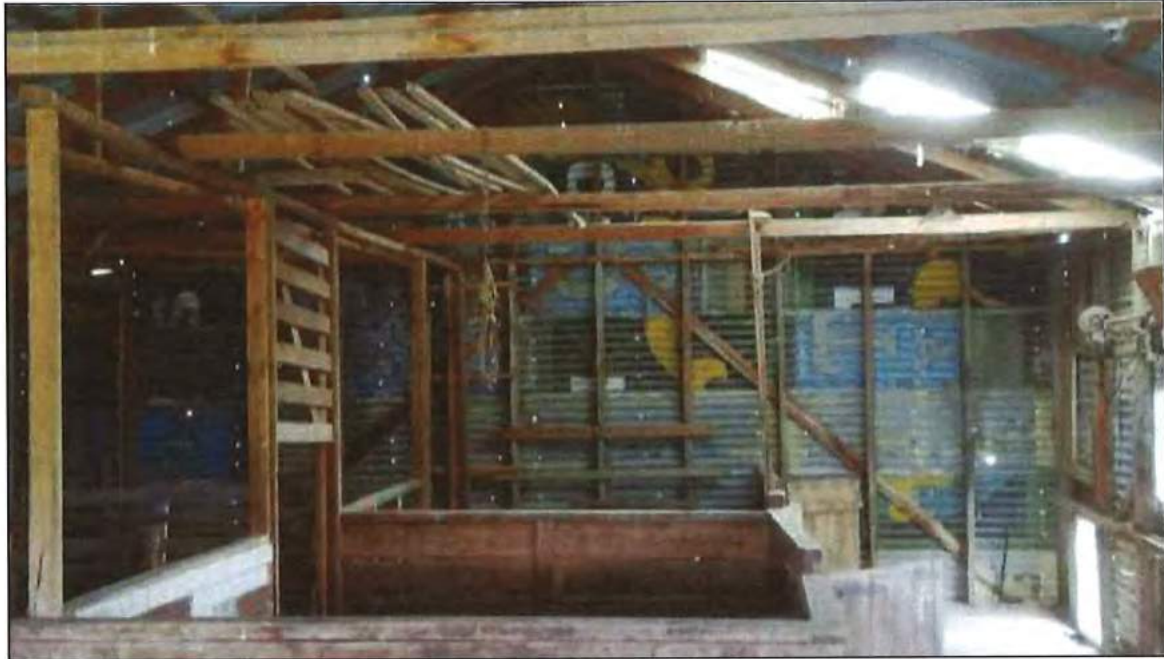
Figure 12. Woolshed interior with recycled corrugate visible, looking north.
