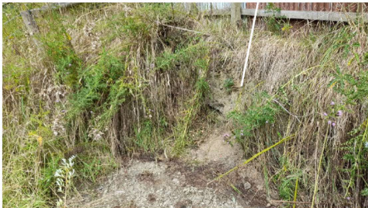
Plate 2: View of the steep excavated slope in the southwest corner of the site.
