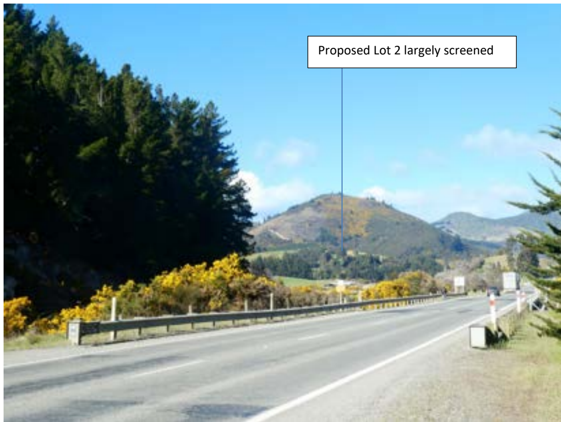
Figure 5: View towards site from SH1 on northern approach
