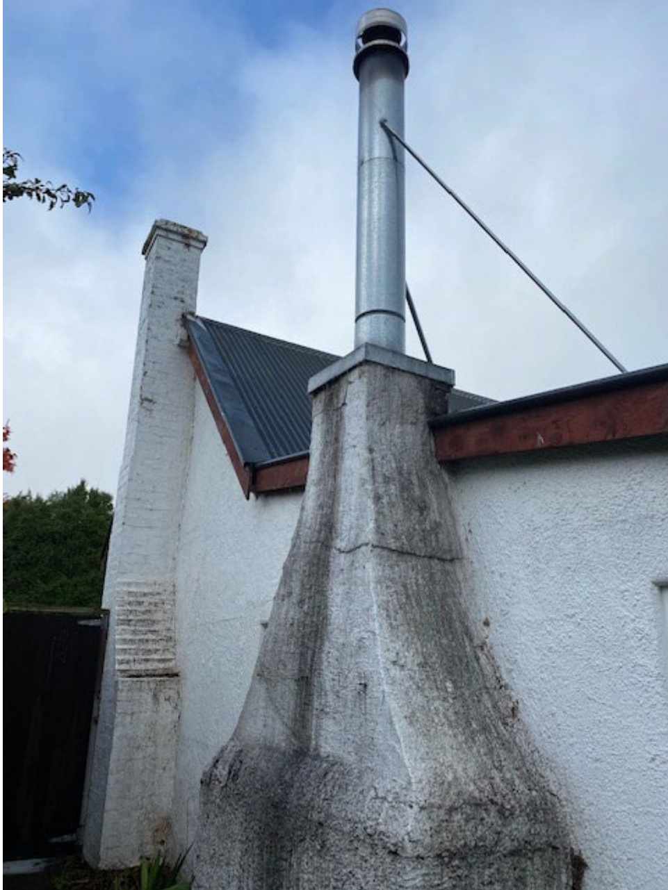
Image 12: Exterior photo of chimneys
