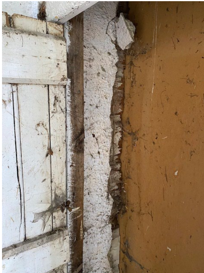
Image 4: Demonstrating Cottage has weatherboard exterior but has been rough cast at a later date.
