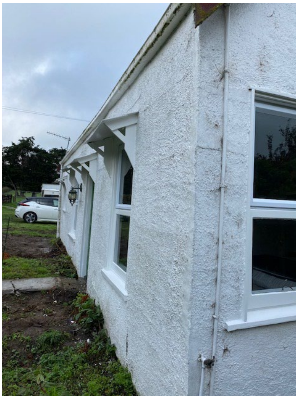
Image 13: Exterior photo of side profile of façade
