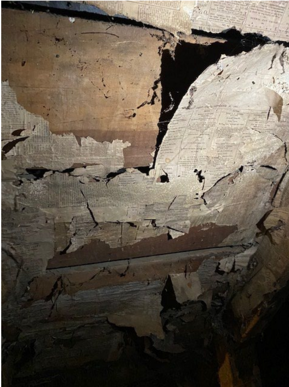
Image 11: Attic: demonstrating old newspaper lining (Otago Witness), proof of habitation
