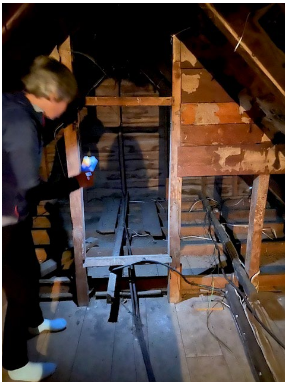
Image 8: Attic: towards wall
