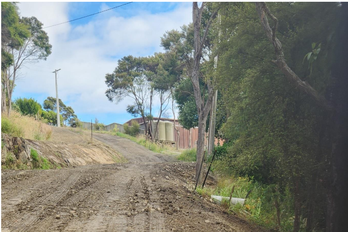
Photograph 5: Re-grading on northern slope now complete (photo supplied by P Napier)
