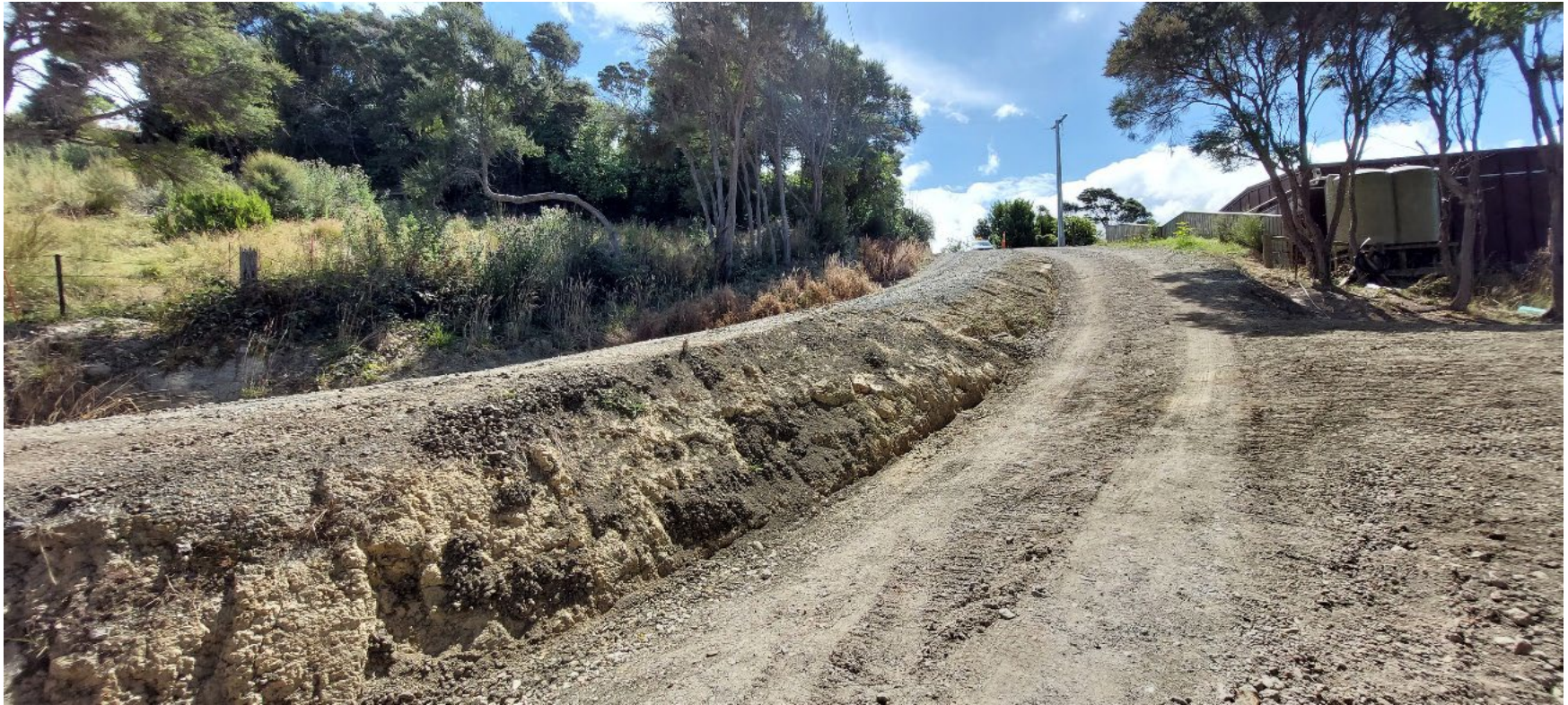
2. Top of old and new access ways, showing cuts. Top part within road reserve is now out of scope
