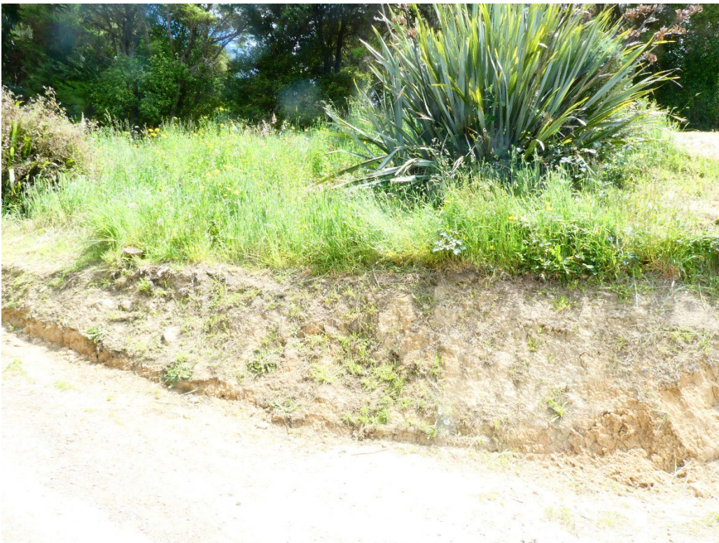
Figure 2: Southern extent of cut slope to be re-battered.
