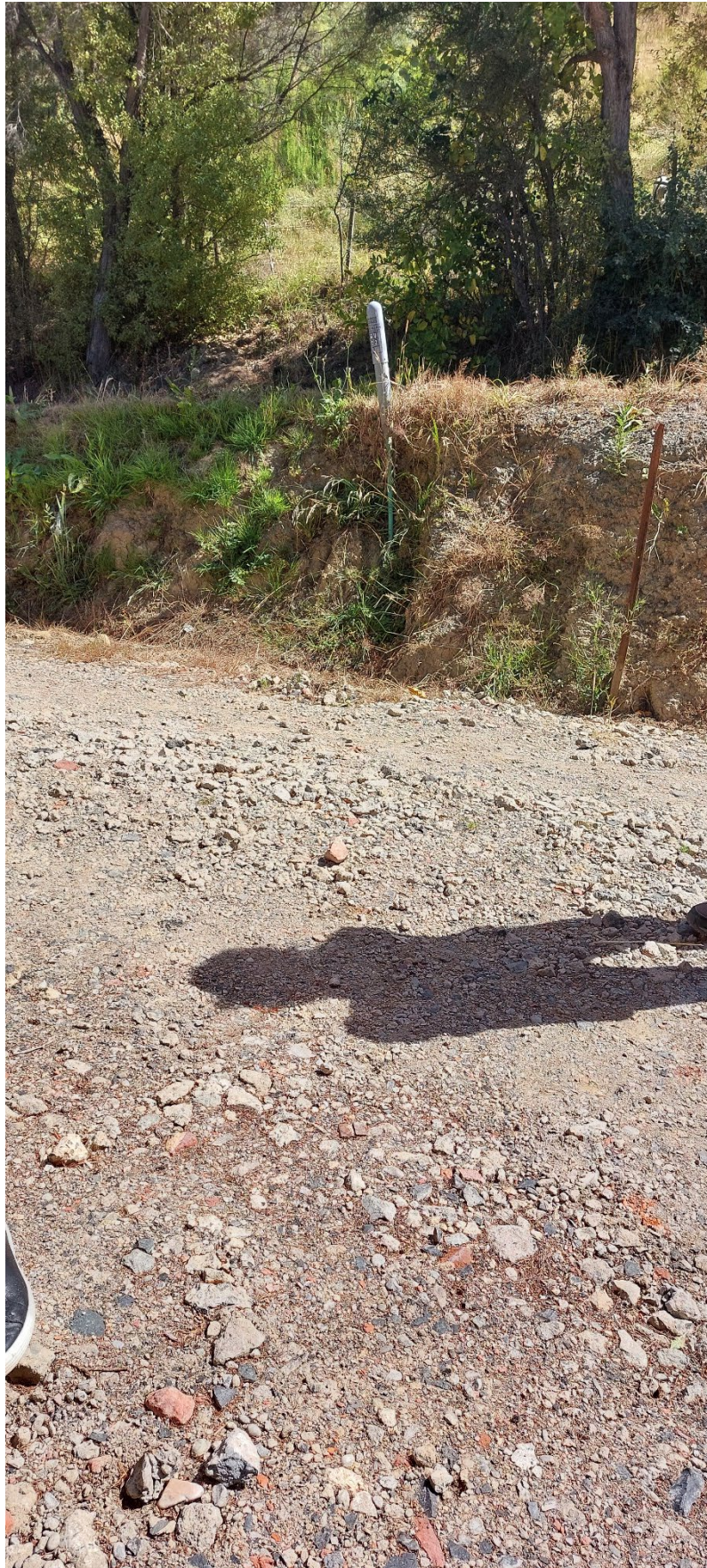
8. Earthworks near telecommunication utility
