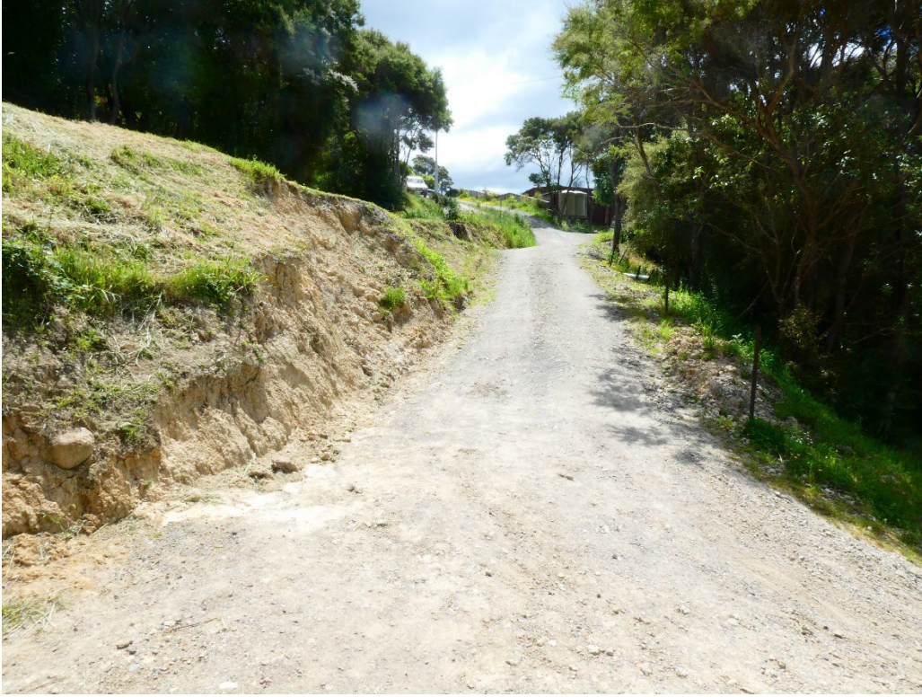
Figure 1: Northern extent of cut slope to be re-battered.
