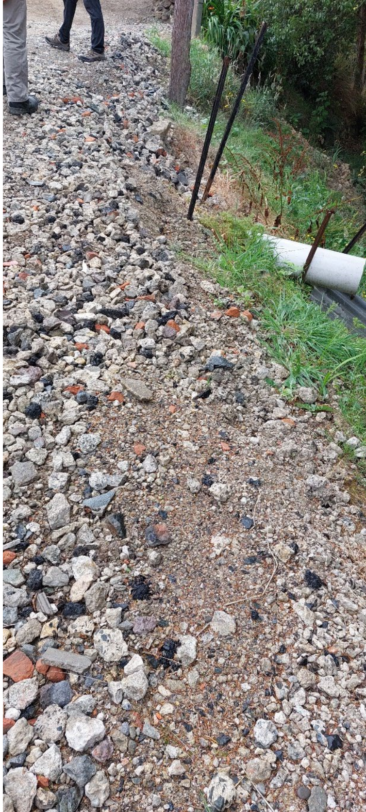
11. New culvert discharge point viewed from above
