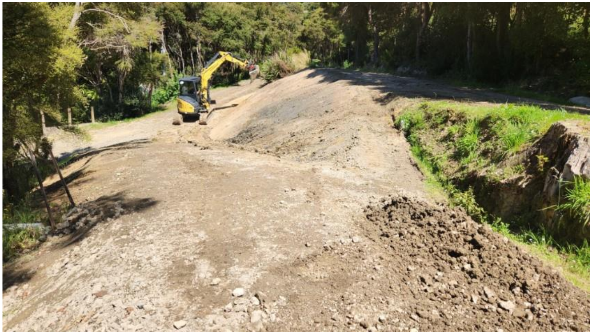
Photograph 4: Main slope at the completion of re-grading (photo supplied by P Napier)
