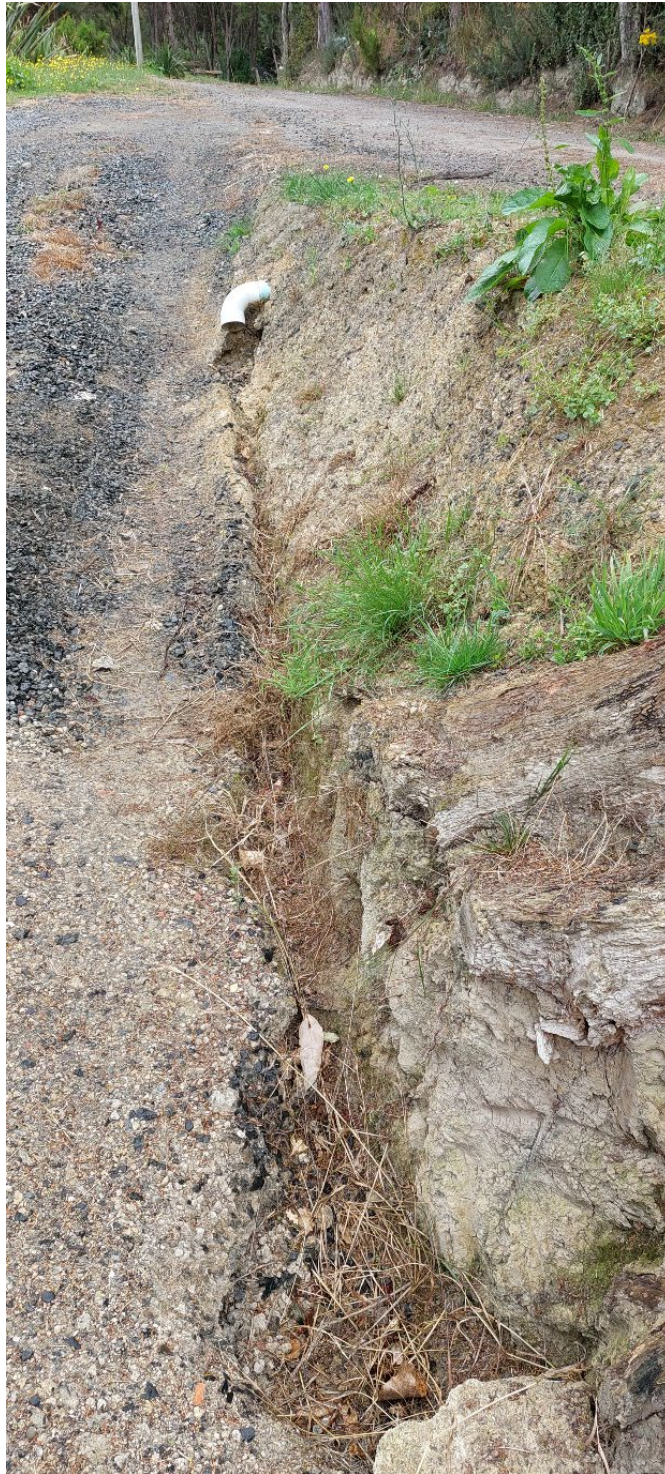
10. Stormwater diverted towards new culvert
