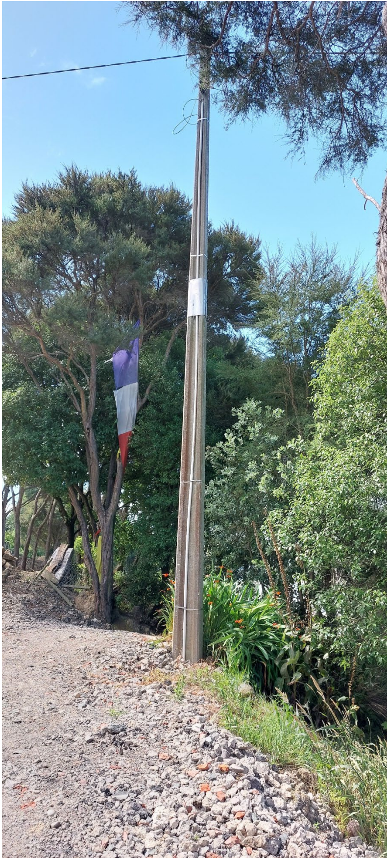
7. Earthworks near electricity pole
