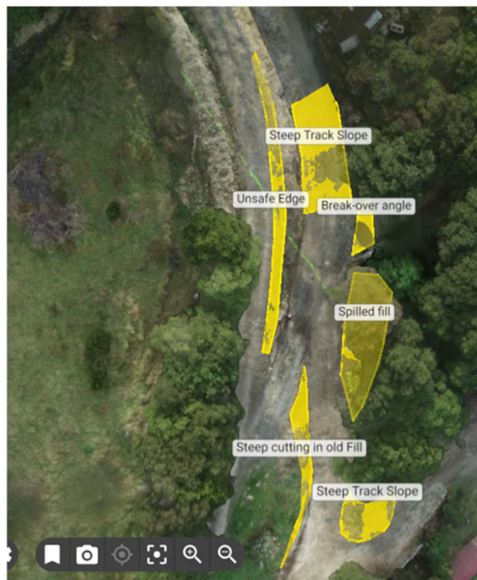
Figure 2: drone image with labels showing 2022 earthworks
