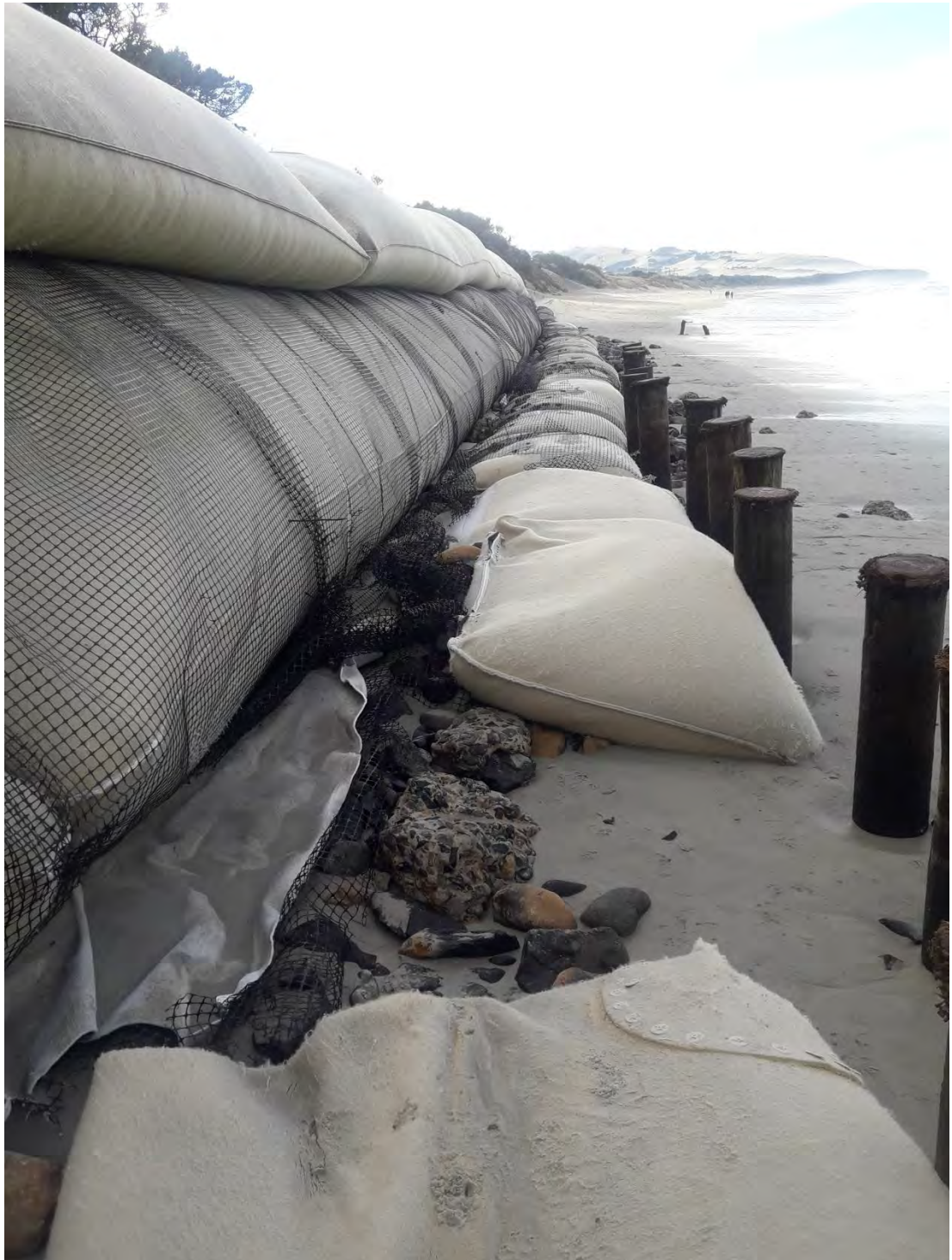
Figure 7.1: Broken geotextile tube on early May 2019 after autumn storm. Photo: Tom Simons-Smith
