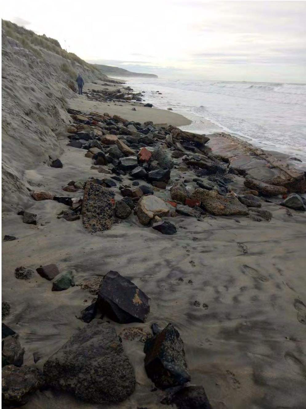
Figure 7.2: Rock and concrete were exposed in front of 4 m dune scarp on Profile 5 of Area 2, after winter storm on early August 2019.
