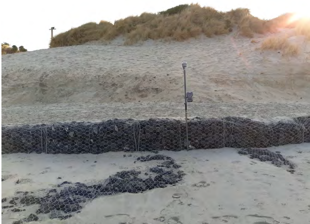
Figure 7.3: Beach erosion of 1 m in Area 2 on the 26 th July 2020.
