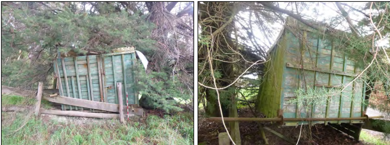
Figure 5-43 Horse float. Note that the roof would normally be flat however the structure is damaged causing the roof to sag in the centre of the side facing the road (left) but remain relatively flat at the opposite side (right). The nails used for the construction of the structure and associated fences appear to be modern.
