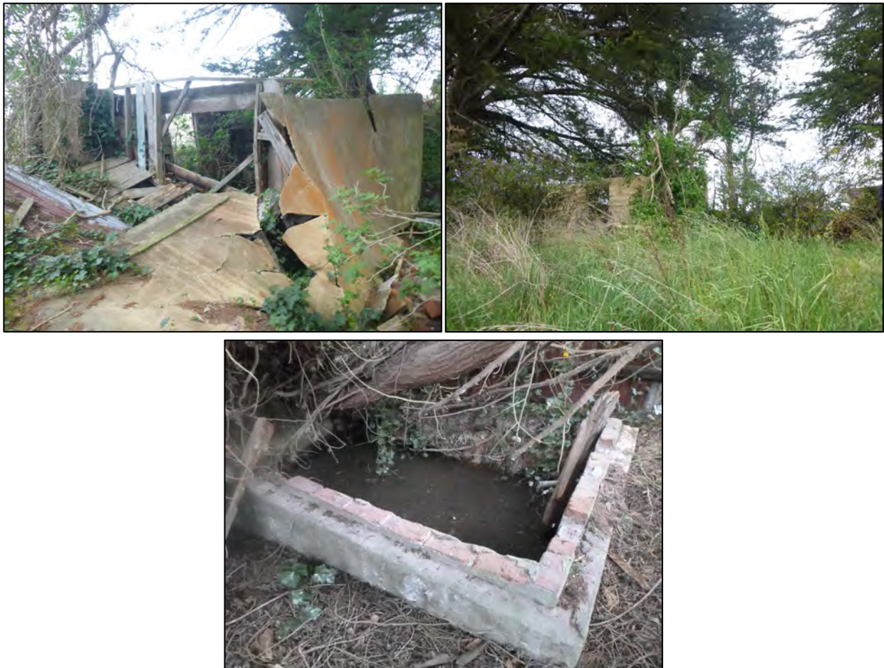
Figure 5-18 Current condition of the homestead structure with the ceiling collapsed and walls listing heavily, looking north (top left) Structure barely visible through thick vegetation, looking south (top right) and the current state of brick and concrete lined structure looking north (bottom).
