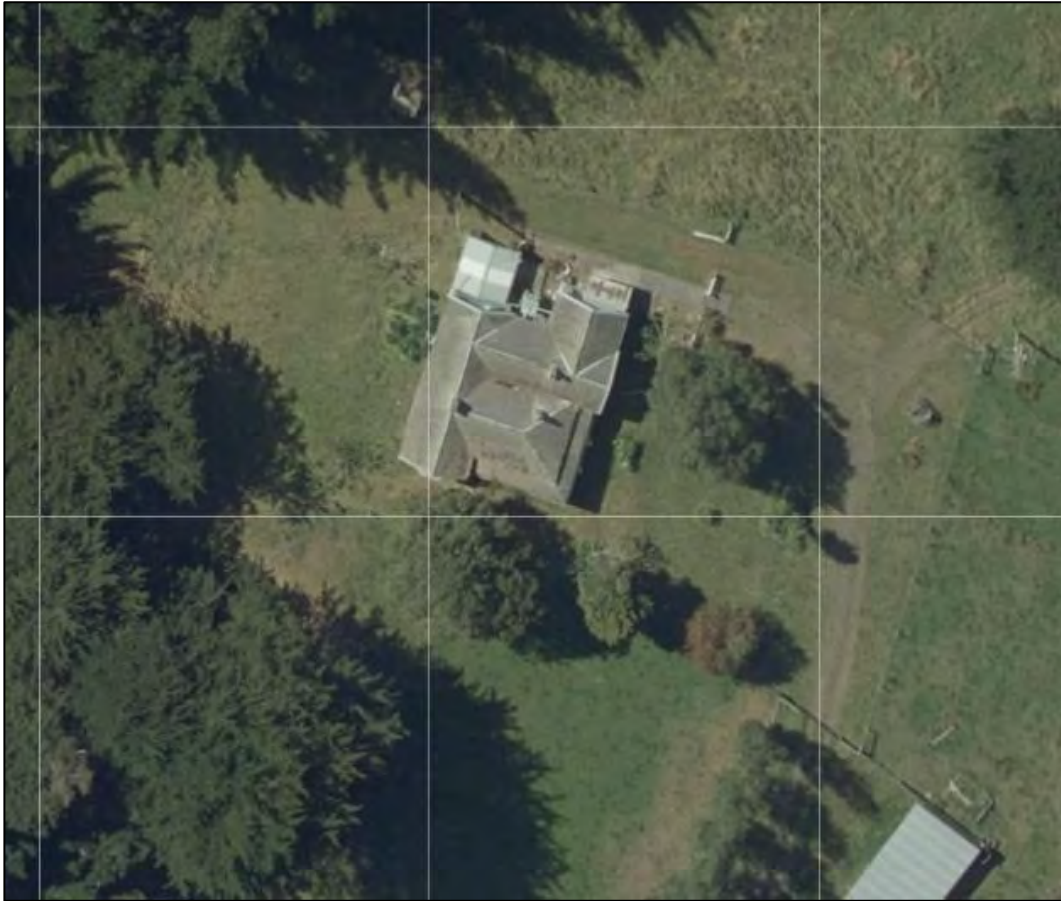
Figure 5- 425-39 2018-2019 aerial showing the pre-1900 building still present on the property today (DCC, Aerial Surveys Ltd, & ORC, 2019).
