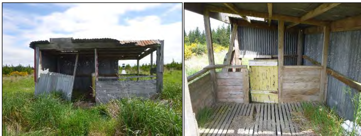
Figure 5-375-34 Site 7 Structure exterior (left) and interior (right).
