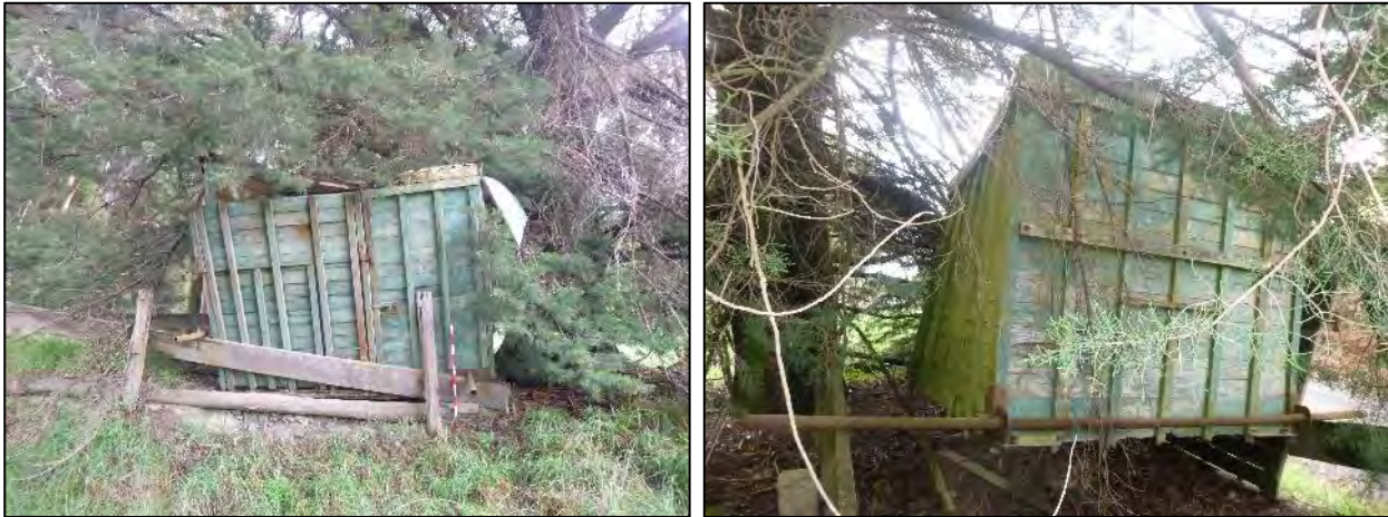
Figure 5-465-43 Horse float. Note that the roof would normally be flat however the structure is damaged causing the roof to sag in the centre of the side facing the road (left) but remain relatively flat at the opposite side (right). The nails used for the construction of the structure and associated fences appear to be modern.
