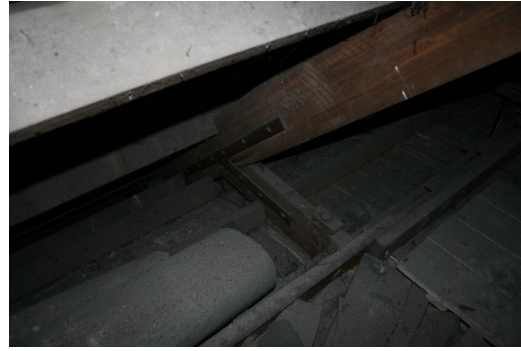
Roof Truss collar tie to rafter connection
