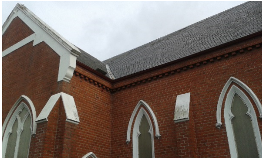
Top of Side walls
