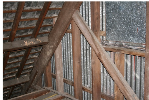
Roof structure at timber gable end wall.
