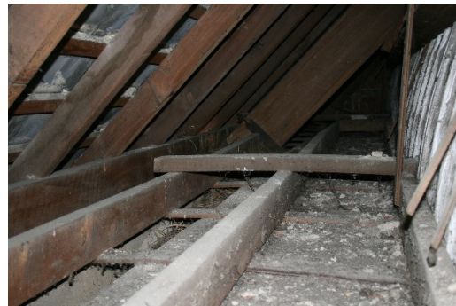
Truss connection to top of brick walls.
