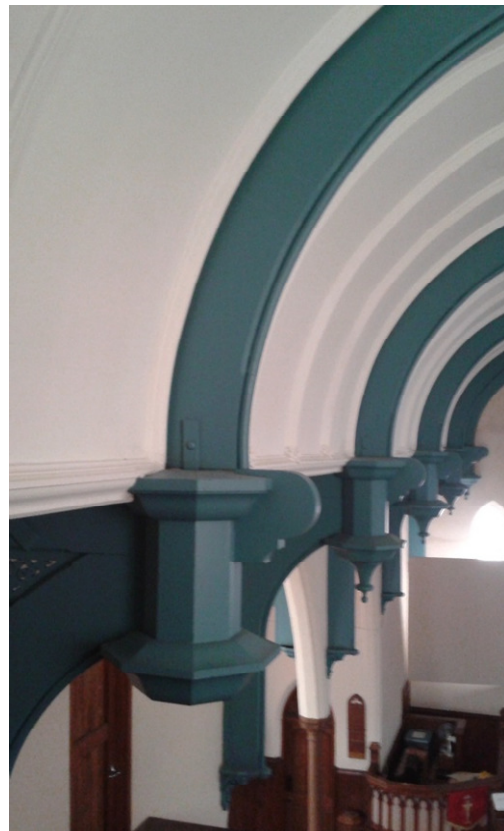
Roof structure detail below ceiling
