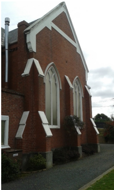
Transept gable end wall
