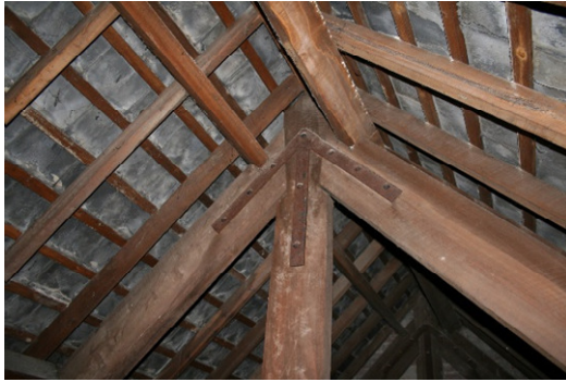
Roof Truss Apex Connection.
