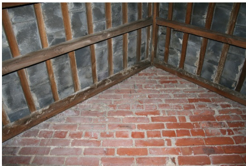
Roof structure at transept gable end.
