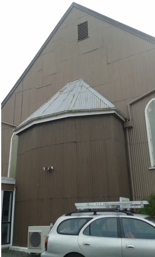
Timber framed gable end wall at SW end of Church
