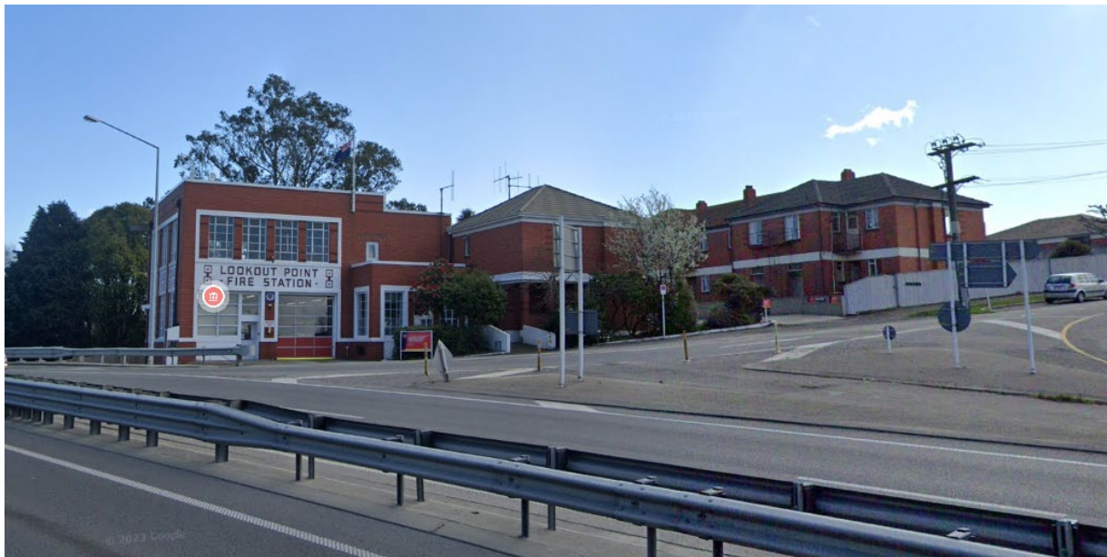
Figure 2: Photograph of the fire station and its accommodation block (Source - Google Maps Sept 2023)
