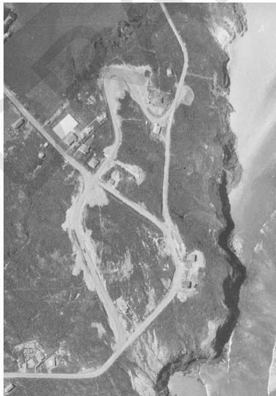
View of Tomahawk Battery, 15 October 1942. Reference: Survey SN223, Run 513, Photo 35. Sourced from http://retrolens.nz and licensed by LINZ. Copyright status: CC-BY 3.0
