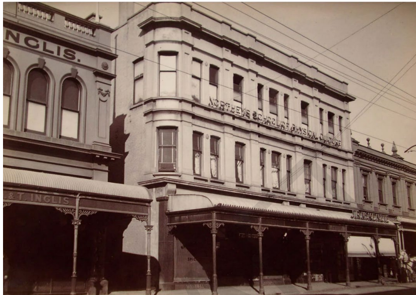
The building showing signage advertising 'Northeys School of Physical Culture' and 'J.R' McKenzie (on the verandah); https://builtindunedin.com/tag/hotels/#jp-carousel-5072
