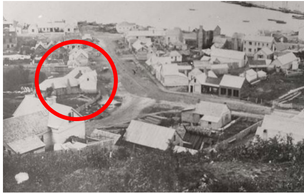
The site prior to the construction of the Hayman & Co. Warehouse. Cropped from Dunedin - early view over Rattray Street, Maclaggan Street, and Otago Harbour (1860s). Hocken Digital Collections, accessed 05/06/2024, https://hocken.recollect.co.nz/nodes/view/43853
