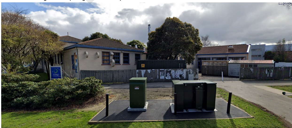
Corner of Albany Street and Anzac Avenue
