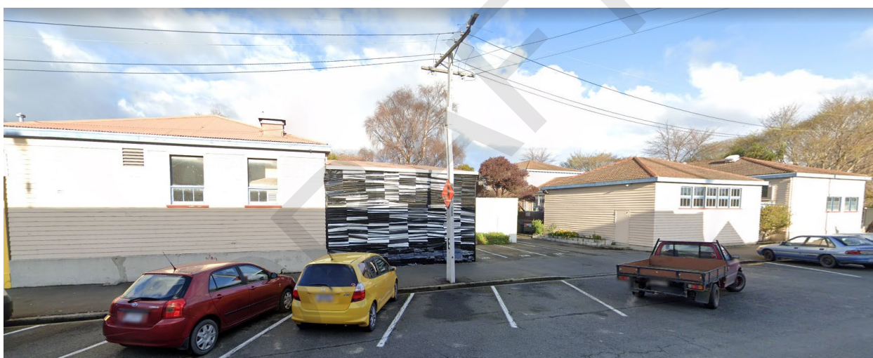
Elevation on Riego Street (Google Streetview)
