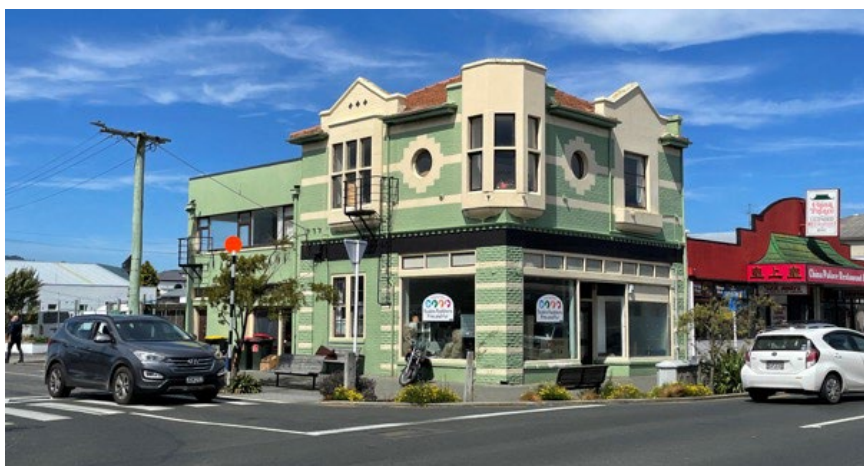
Photograph: DCC, October 2022
