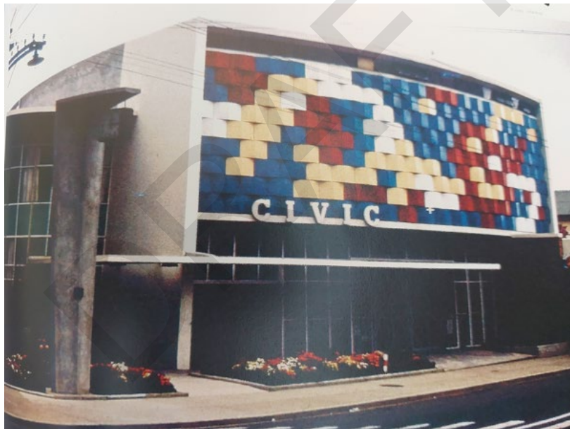
Civic Centre before repainting (The Allingham File compiled by Nigel Brown)
