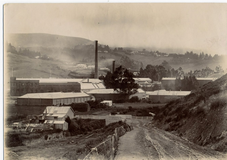
Undated image of the mills from Stone Street (Toitū 58_14-1)
