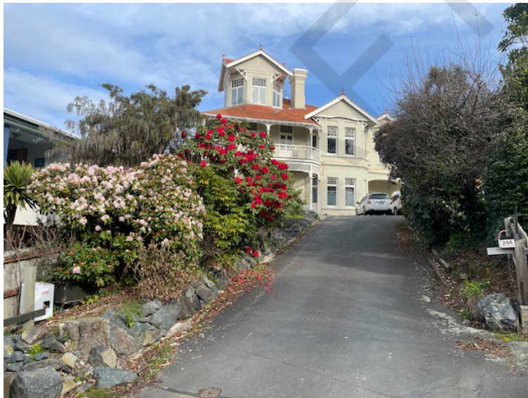
View from the bottom of the driveway
