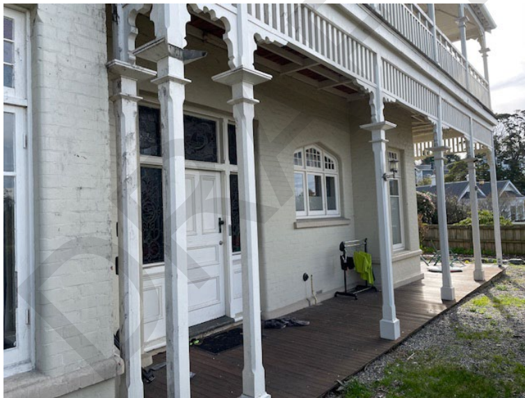
The main entry door opposite the top of the stairs in the following image. Source: DCC
