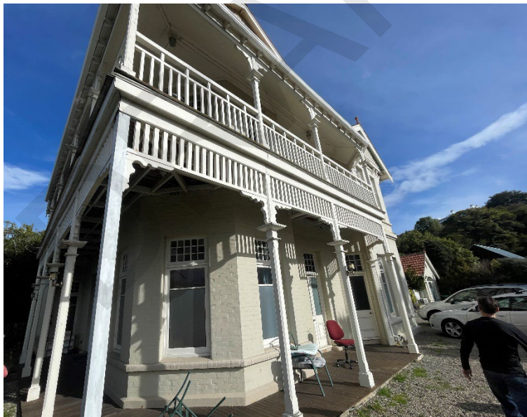
The northeast corner of the dwelling showing the verandah. Source: DCC
