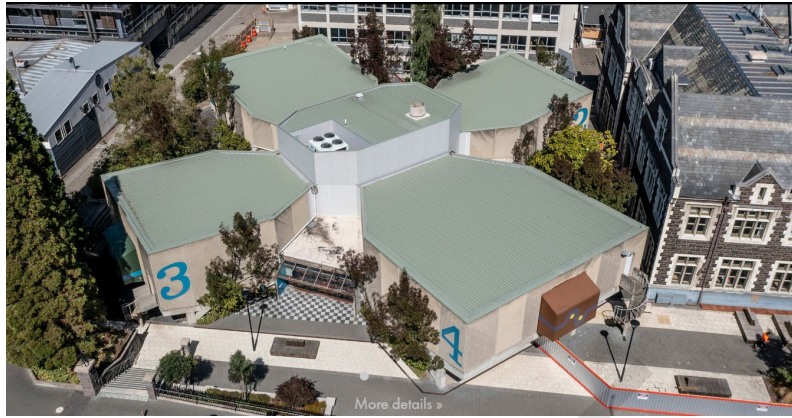
ARCHWAY LECTURE THEATRES | McCoy Wixon Architects
