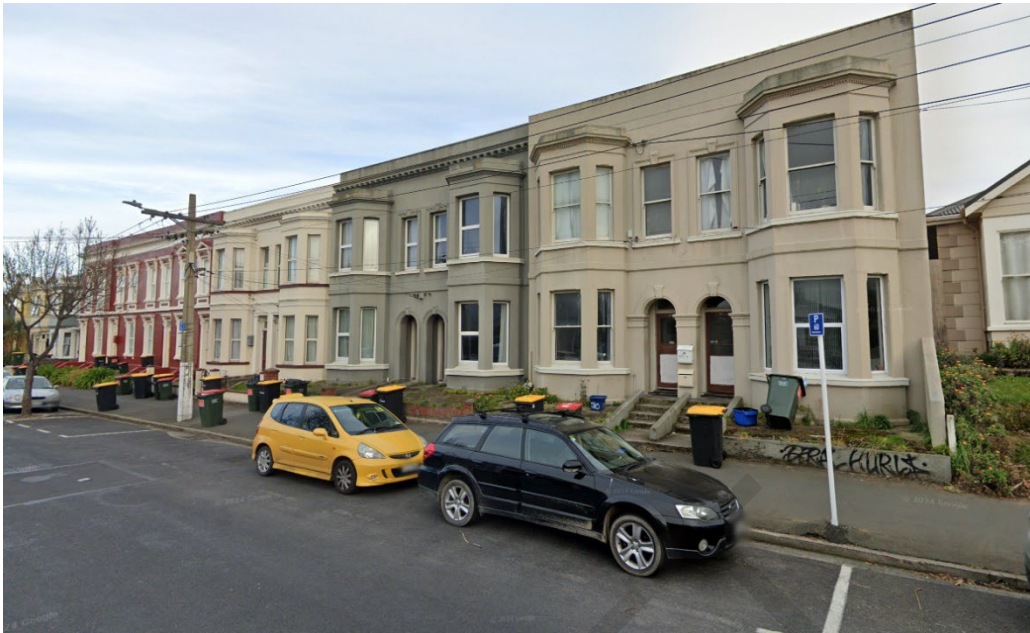
Streetscape context, Google Street View
