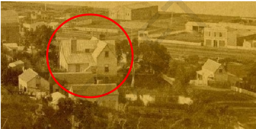
Toitu 65_37-1 – prior to 1870- 1875 (first church under construction)
