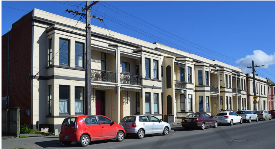
Photograph: Built in Dunedin
