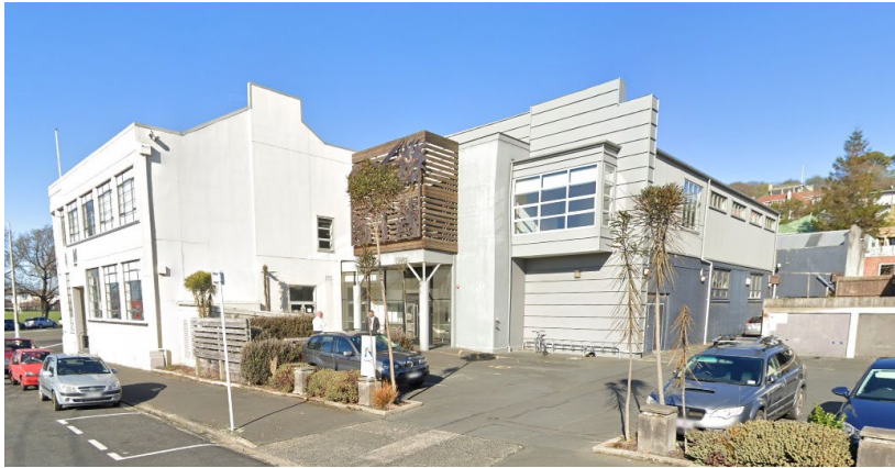
Additions to Melville Street elevation. Google Street view (2020)
