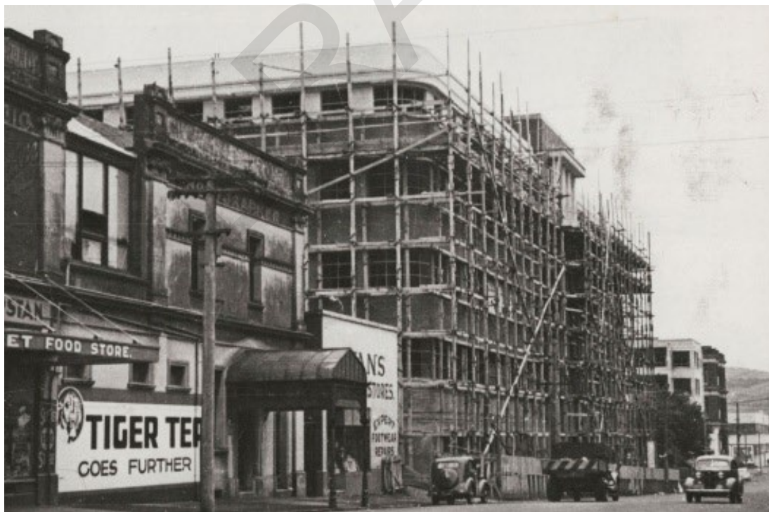
The new south block under construction. Hocken Collections, University of Otago.
