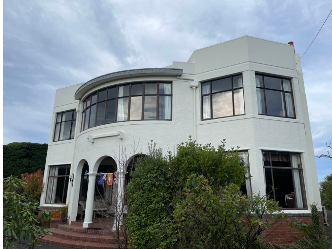
The principal northwest elevation
