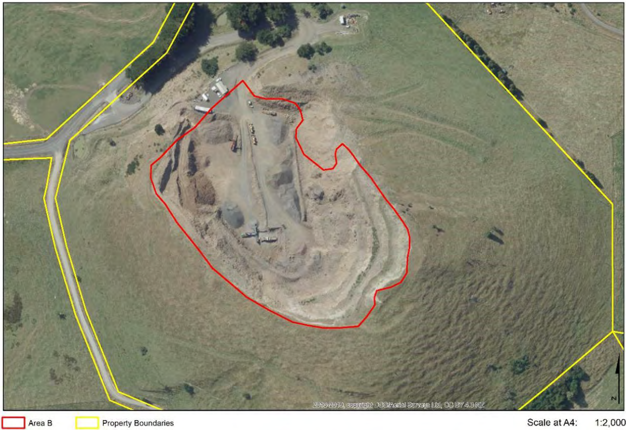
Figure 16.5.16.4B: Saddle Hill Lower Quarry: Operating Limits
