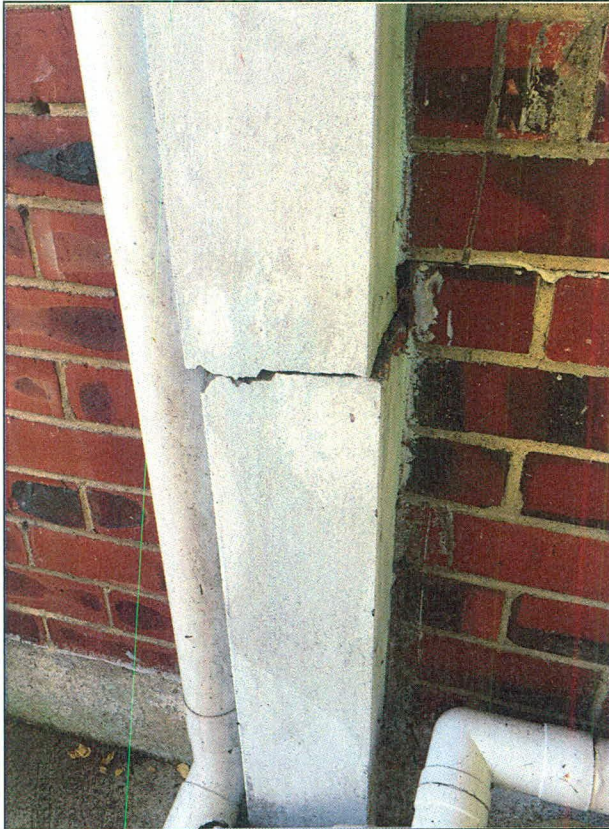
West Fall – masonry movement joint- service box
