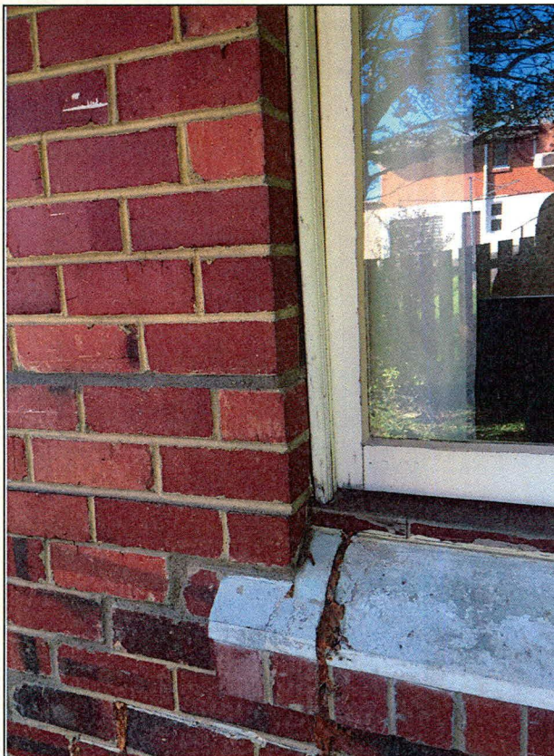
West Fall – Right Window – corner crack – left sill separation
