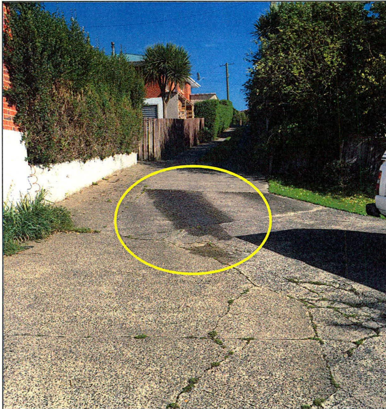
Driveway showing discharge of drains to surface
