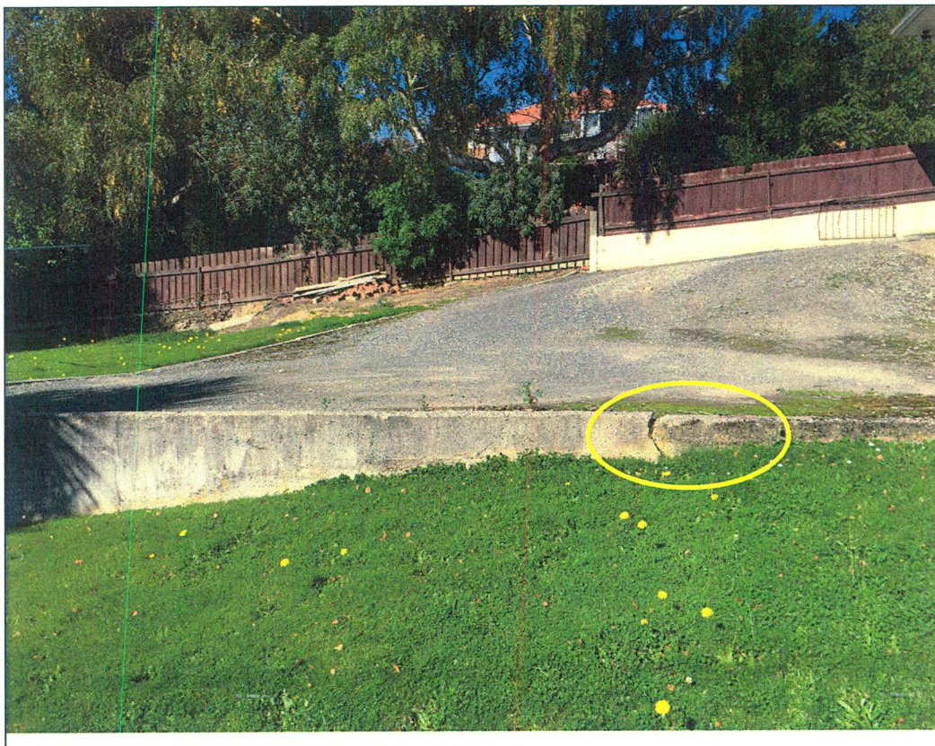
Rear platform to 239 Brockville – separating concrete wall.
