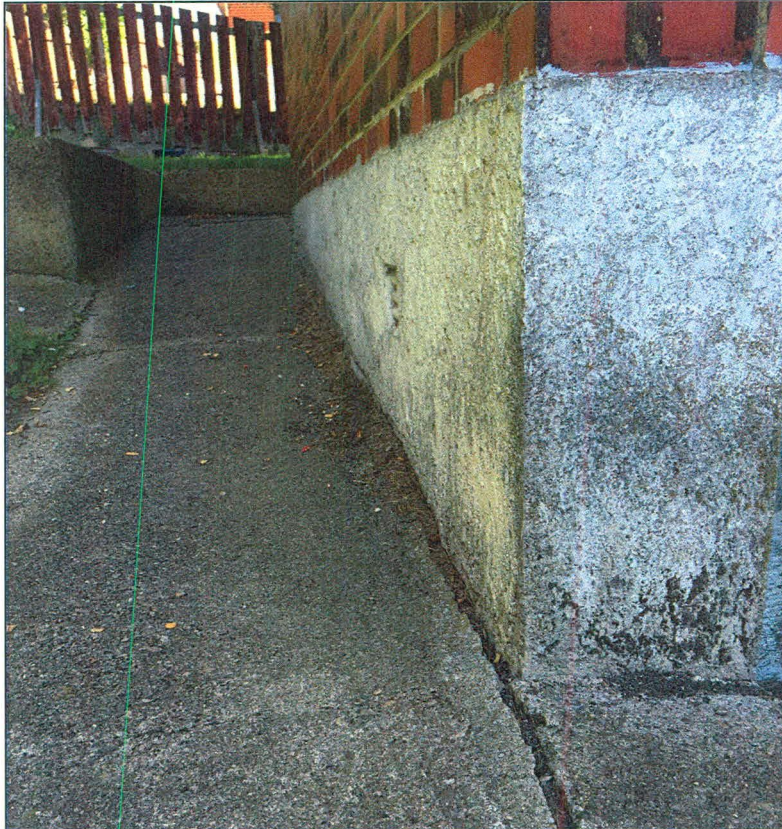
SE Corner – path separation
