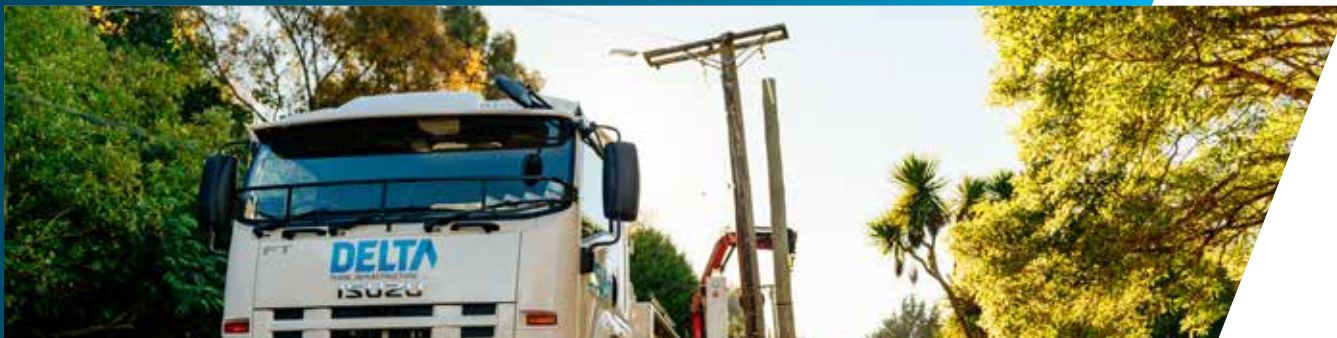
Pole replacement on the Aurora Energy electricity network
