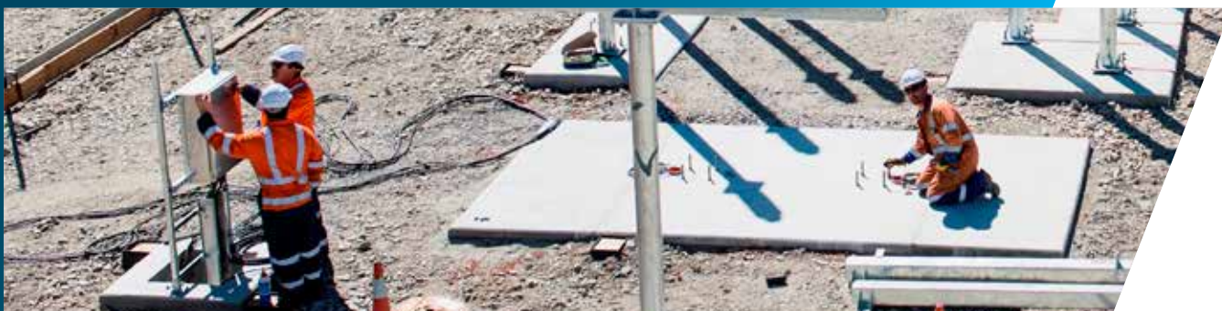
Construction of Lindis Crossing substation, Central Otago
