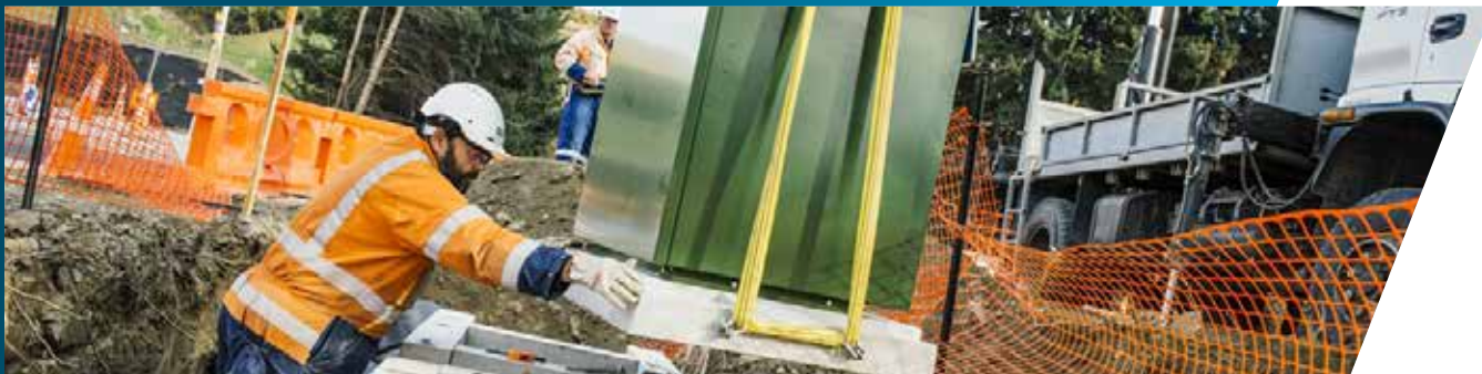
Installing switchgear at Five Mile, Queenstown
