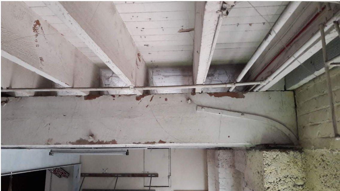
Figure 9 – Tongue and groove floor on 300mm x 45mm timber joists on timber flitch beam. No visible connection from flitch beam to concrete cap on pilaster.
