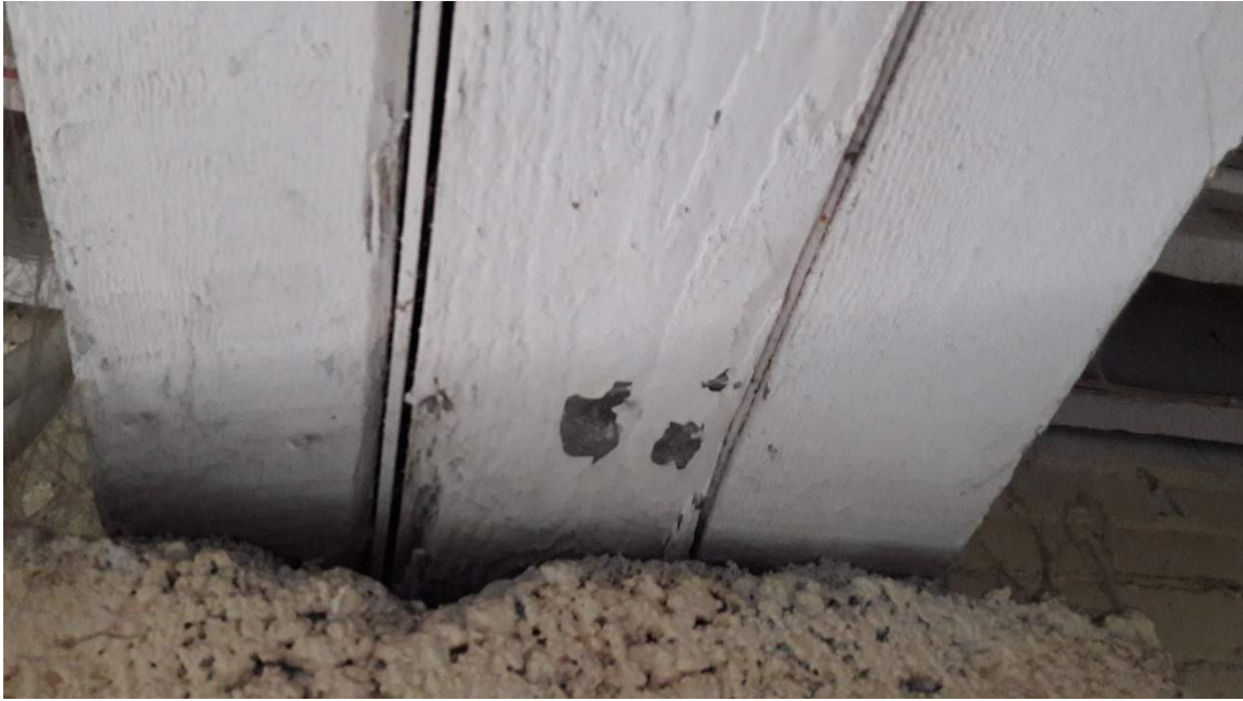
Figure 10 – Timber flitch beam in basement, consisting of 3x 400mm x 150mm timbers and 2x 6mm steel plates.
