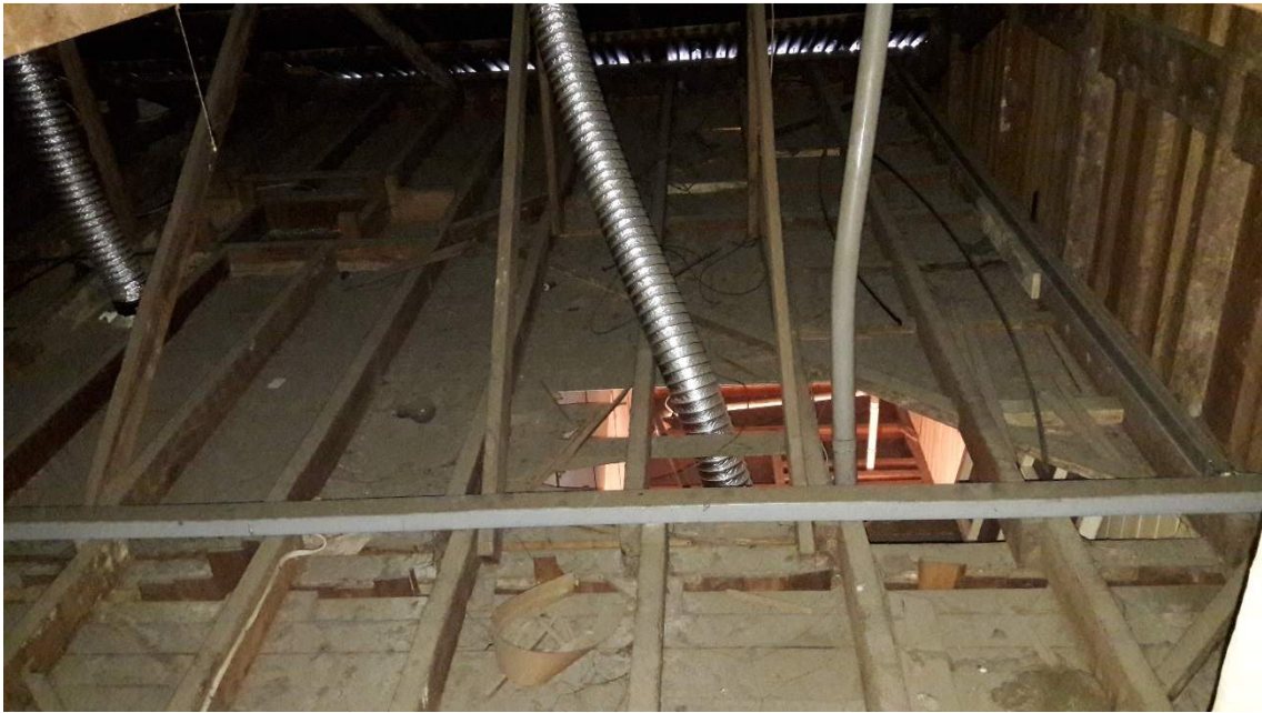
Figure 8 – 130mm x 50mm ceiling joists supporting tongue and groove ceiling lining. Penetration for services down to lower ceiling in ladies' toilets.
