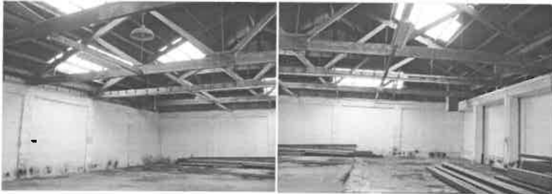
roof trusses on concrete frames and URM walls
