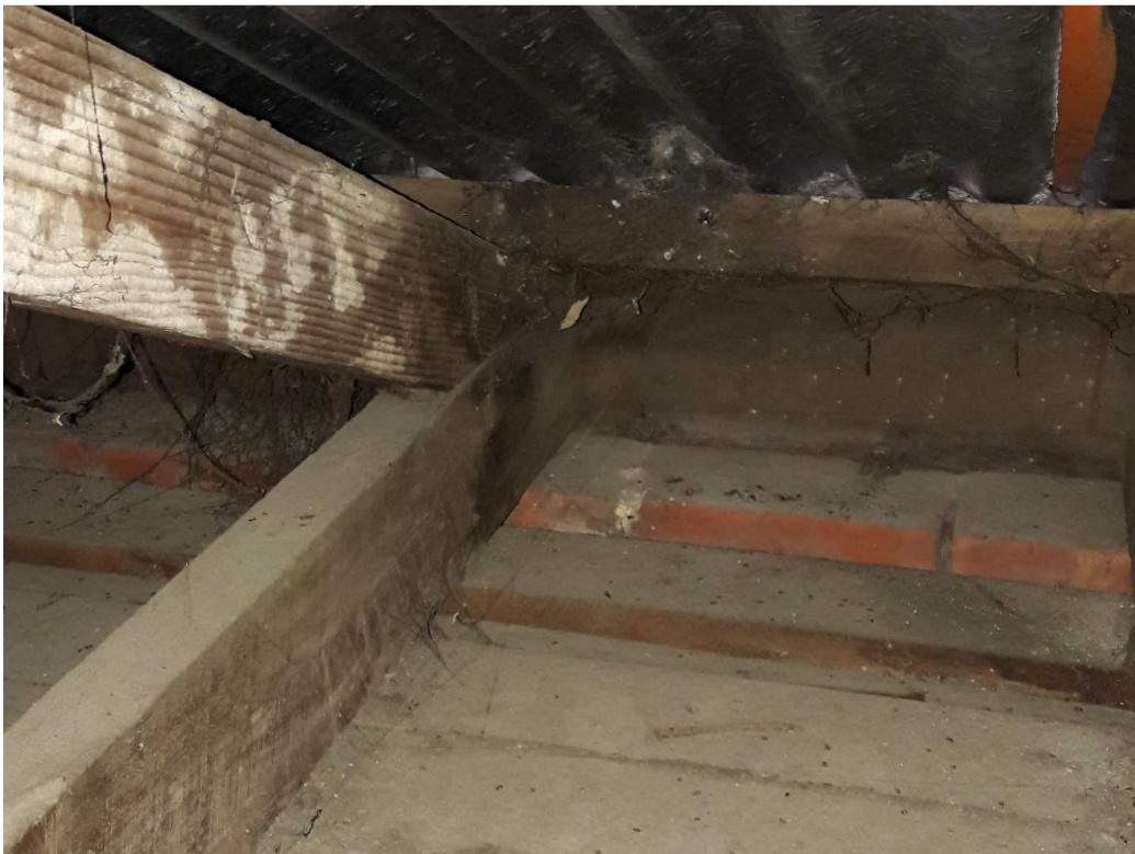
Figure 7 – 100mm x 45mm roof rafter sitting on wall in south end of building. Note no fixing between rafter and wall.
