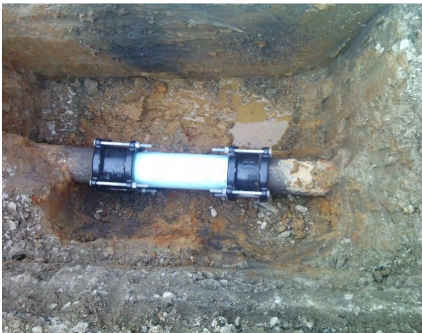
Figure 3-1 Repair to the 'Leak' that occurred in February 2015, photo courtesy Dunedin CC
