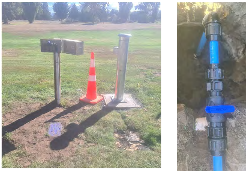
Figure 30: (a) Plastic Sample Station (left) and Steel (right) @ 210 Edinburgh St (also installed at Bendigo Rd.) (b) Plastic tap connection to main
