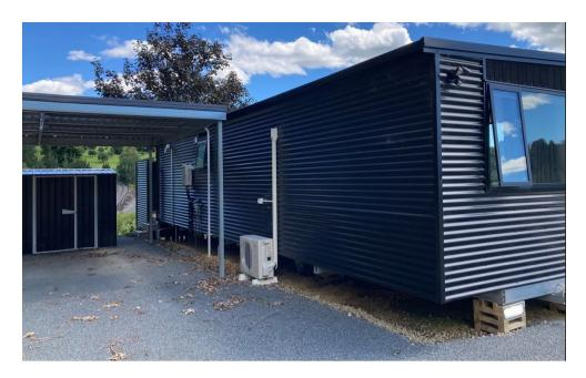
This tiny home is a vehicle with trailer features but is not moveable due to external heat pump unit. It may be considered to be a building if occupied by people on a permanent or long-term basis and **building consent is required**.
