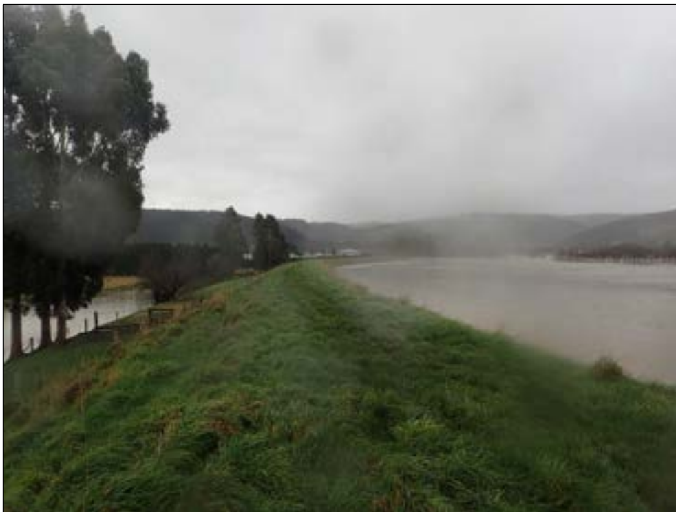
Photograph 1: View North Along Flood Bank (2017 Flood Event)
