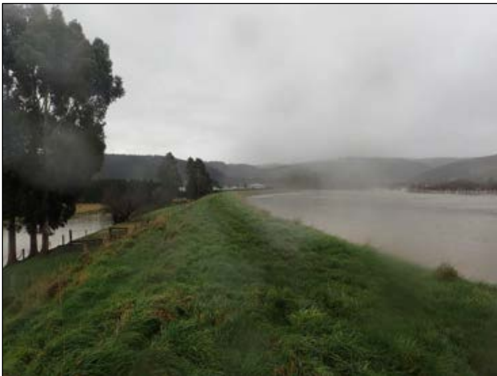
Photograph 1: View North Along Flood Bank (2017 Flood Event)
