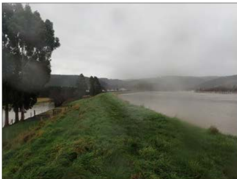
Photograph 1: View North Along Flood Bank (2017 Flood Event)
