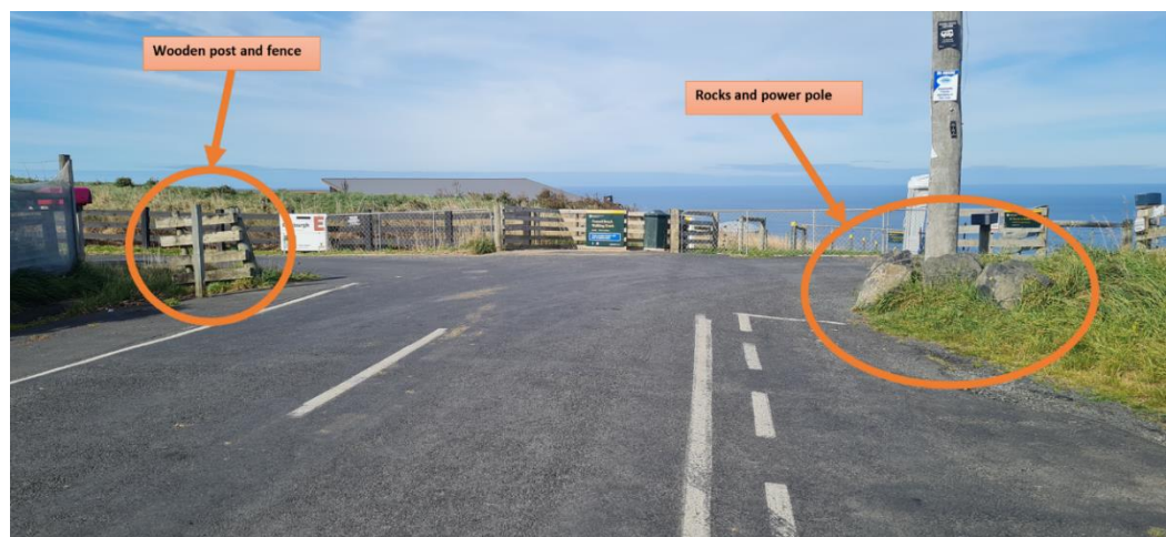
Figure 1: Constraints that impact vehicle tracking into existing accesses
