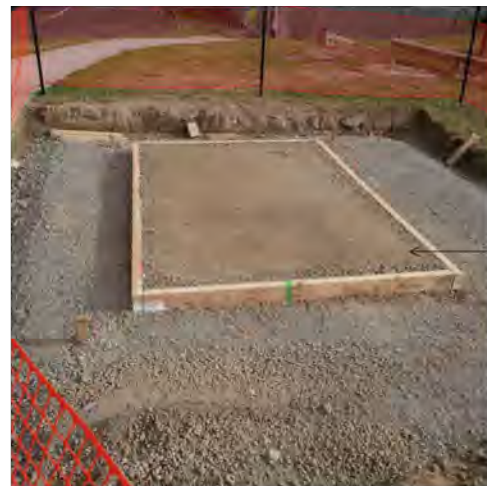
Image showing unit base contained within permanent formwork filled with compacted hard fill and ready for unit to be lowered into place.
