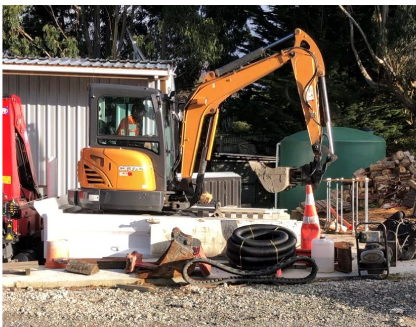
Figure 1: Excavator driving off truck
