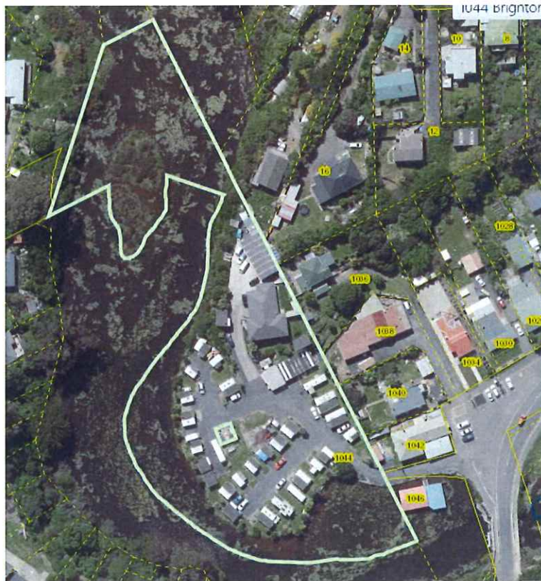
Figure 1: Aerial photograph of 1044 Brighton Rd. Note parcel in centre of site containing Dunedin City Council wastewater pumping station (source: Geocortex).
