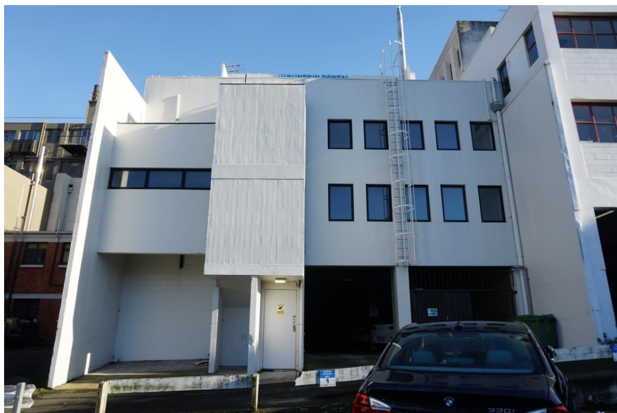
Building F, 169 Princes Street
