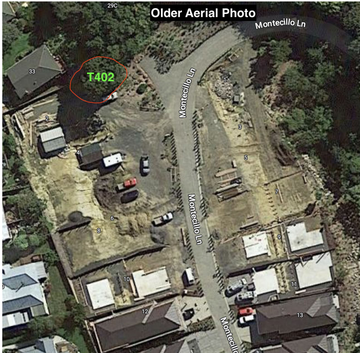
Figure 2: An aerial photo taken during the construction of the new subdivision on Montecillo Lane. Note the reduction in the canopy of T402 compared to figure 1 and the earthworks within its vicinity.
