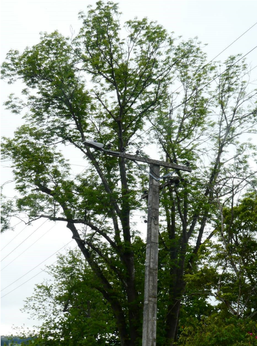
Figure 3. Close proximity view of T1191.
