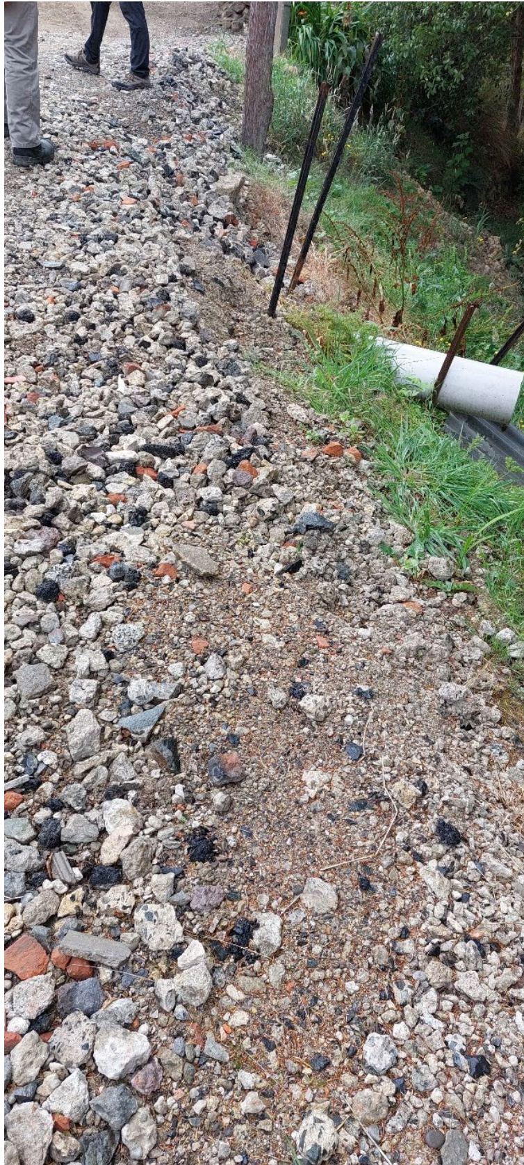
11. New culvert discharge point viewed from above
