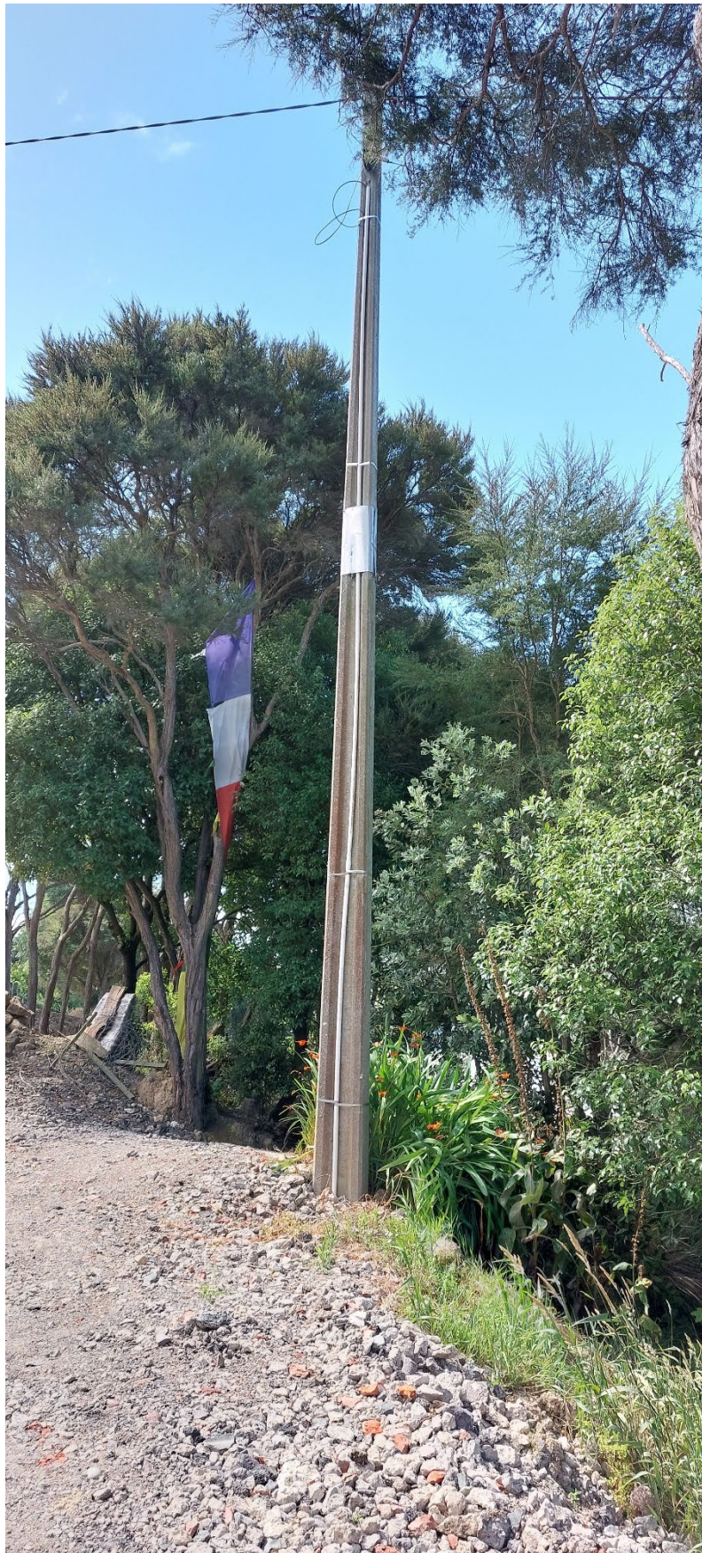
7. Earthworks near electricity pole
