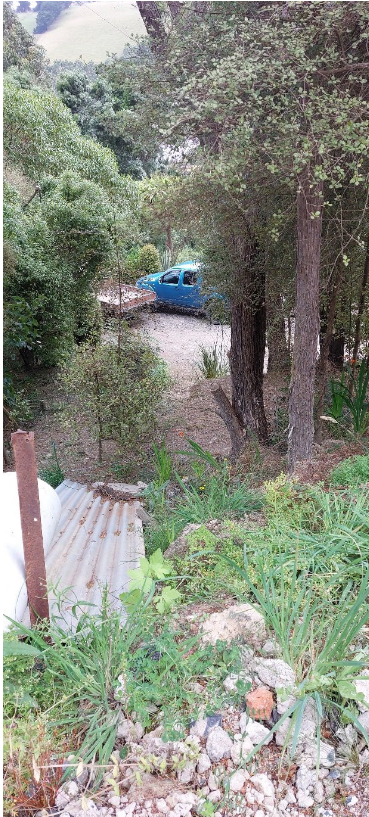
12. New culvert discharge point viewed from above
