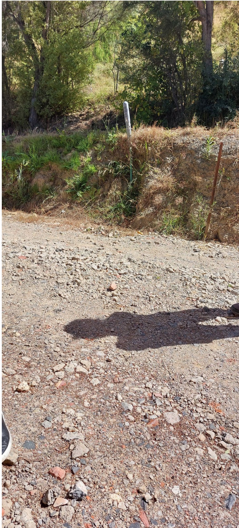
8. Earthworks near telecommunication utility
