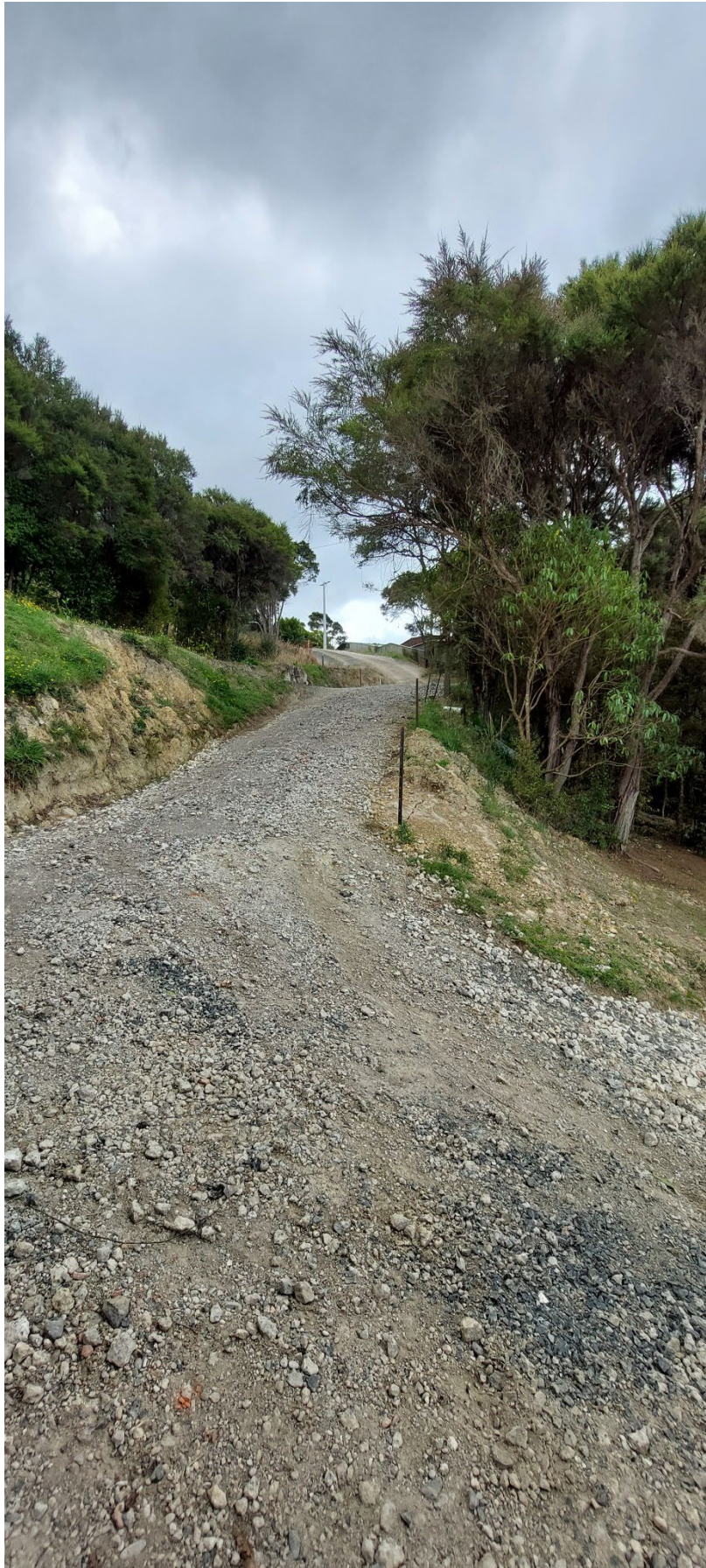
3. New access way viewed from Annie St below
