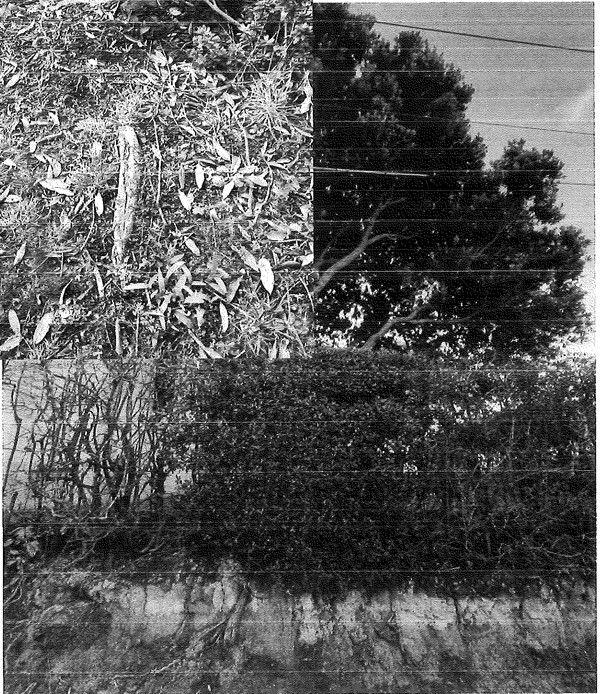
Severed exposed roots – South side clay bank
